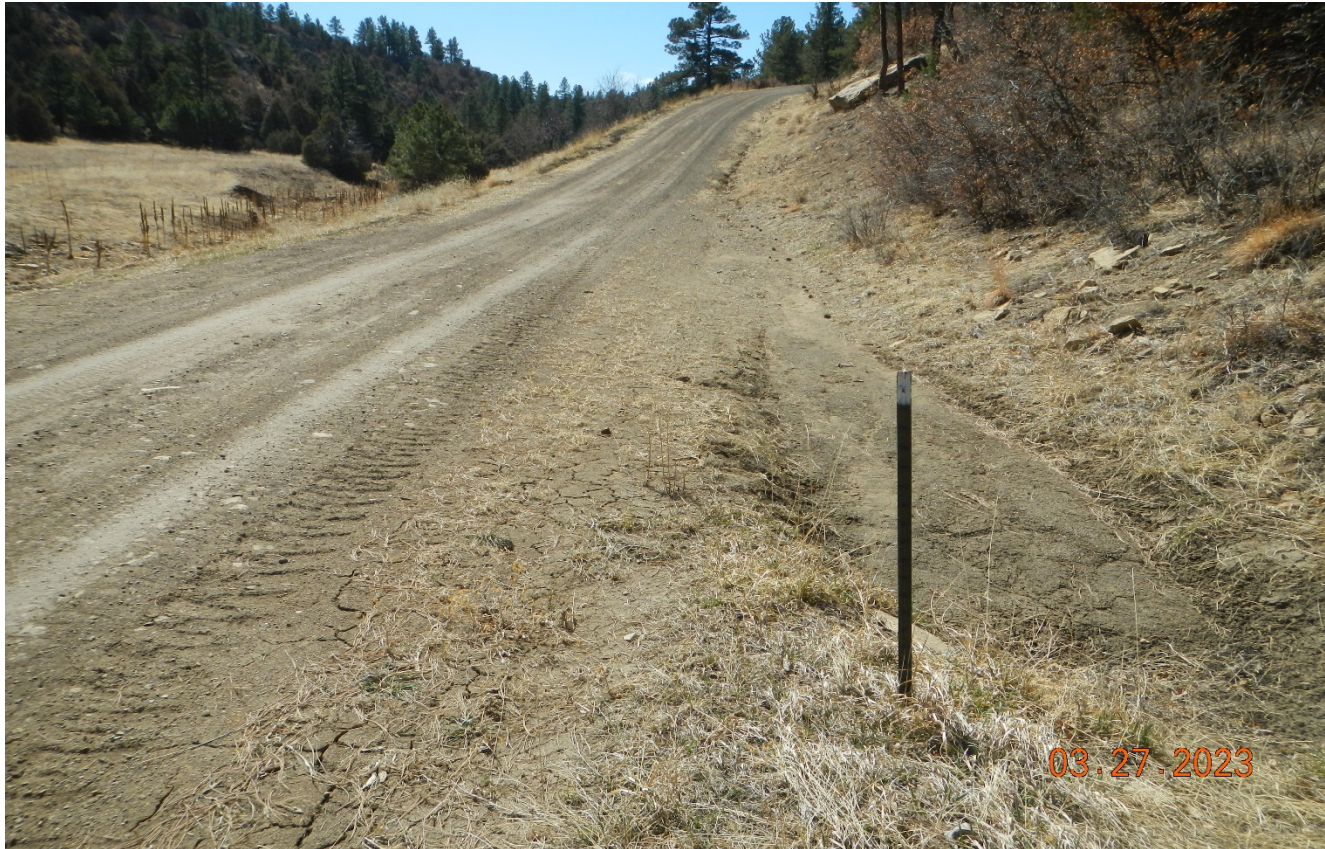
Photo 2. Facing southeast along the access road. This culvert along the access road has filled back in with sediment and needs to be cleaned out.
