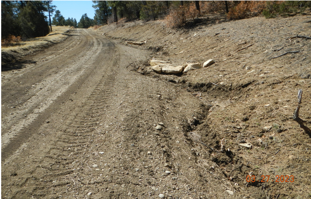
Photo 3. There was repairs made since previous inspection however erosion is occurring around the rock check dams. BMP maintenance is needed.
