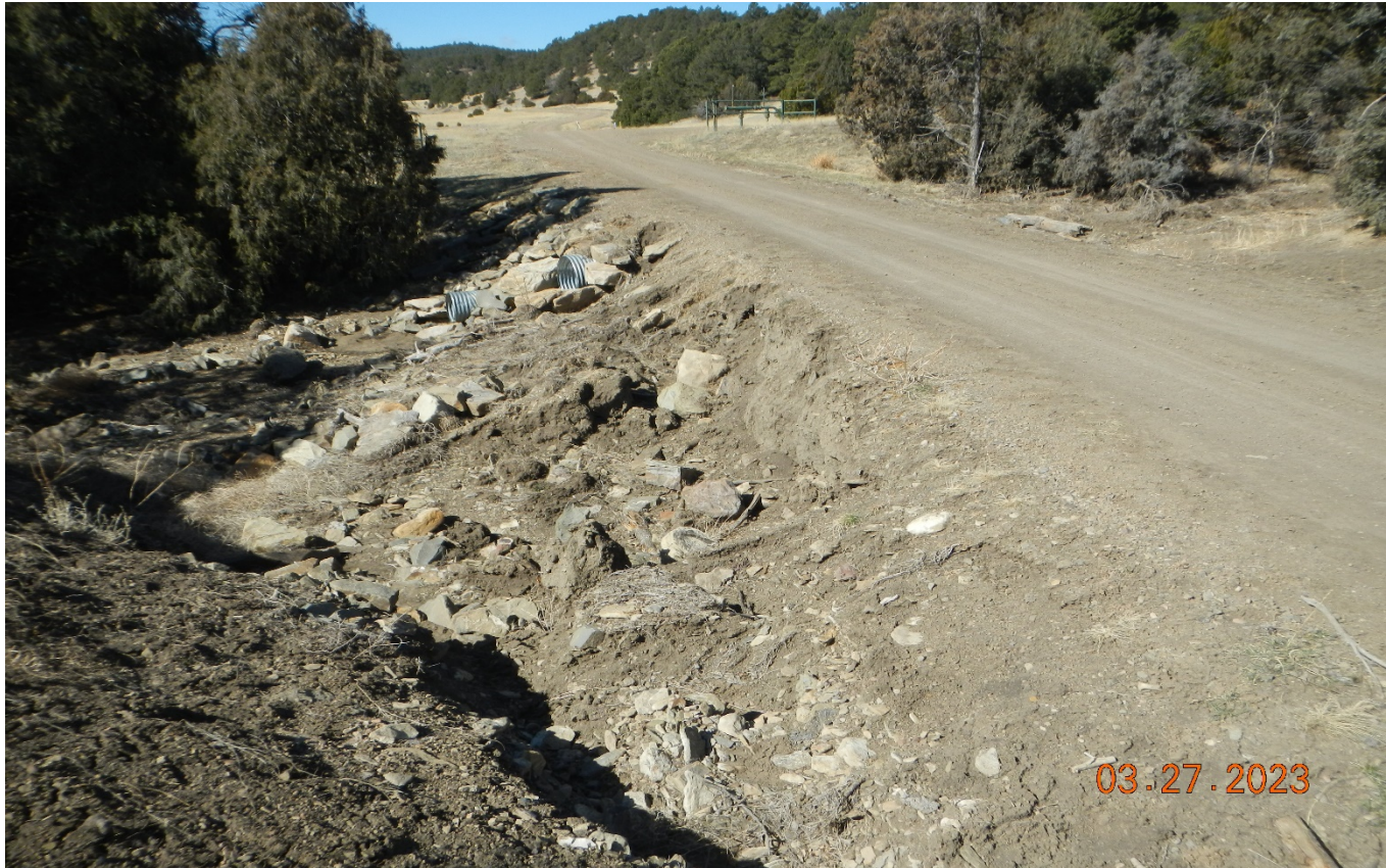
Photo 1. There is erosion along the access road at this drainage crossing Lat/Long:37.05023,-104.66580. This embankment needs to be stabilized.
