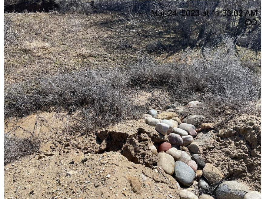
Photo # 3173 Berm & Rip Rap need maintenance/transport of sediment off location
