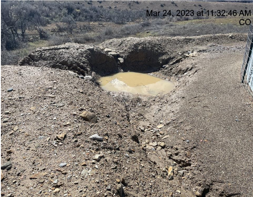
Photo # 3172 Ditch & sediment trap need maintenance
