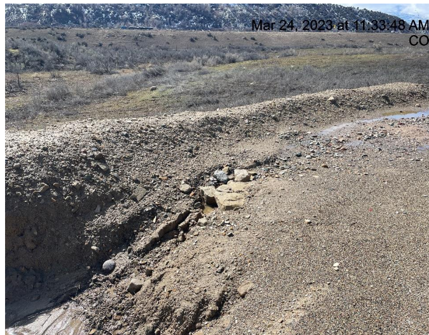
Photo # 3176 Sediment trap/rip rap need maintenance
