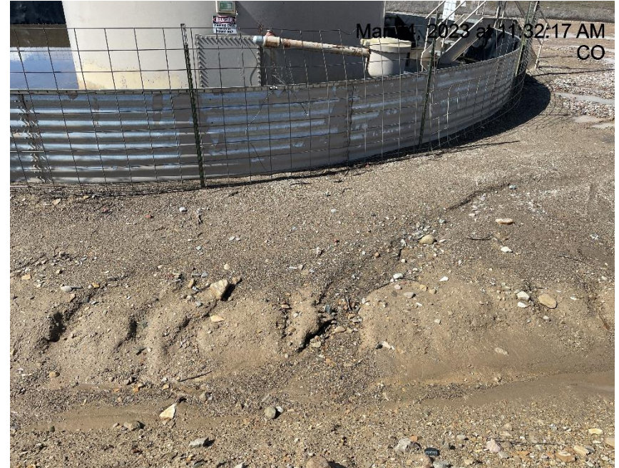
Photo # 3170 Rill erosion
