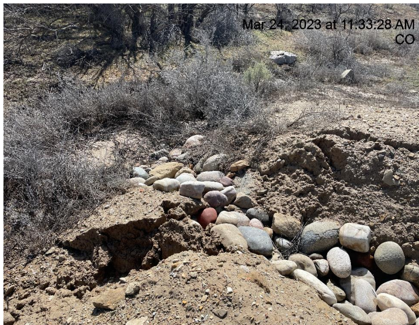
Photo # 3174 Berm & Rip Rap need maintenance/transport of sediment off location
