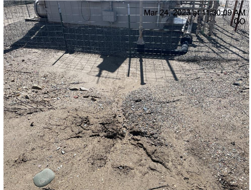
Photo # 3165 Rill erosion/sediment encroaching on equipment
