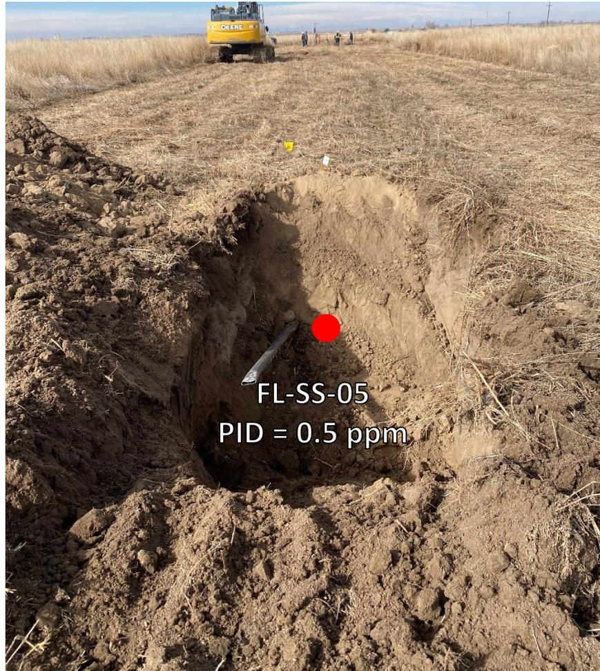
Looking west at bellhole/cut-point for removal – field screened
