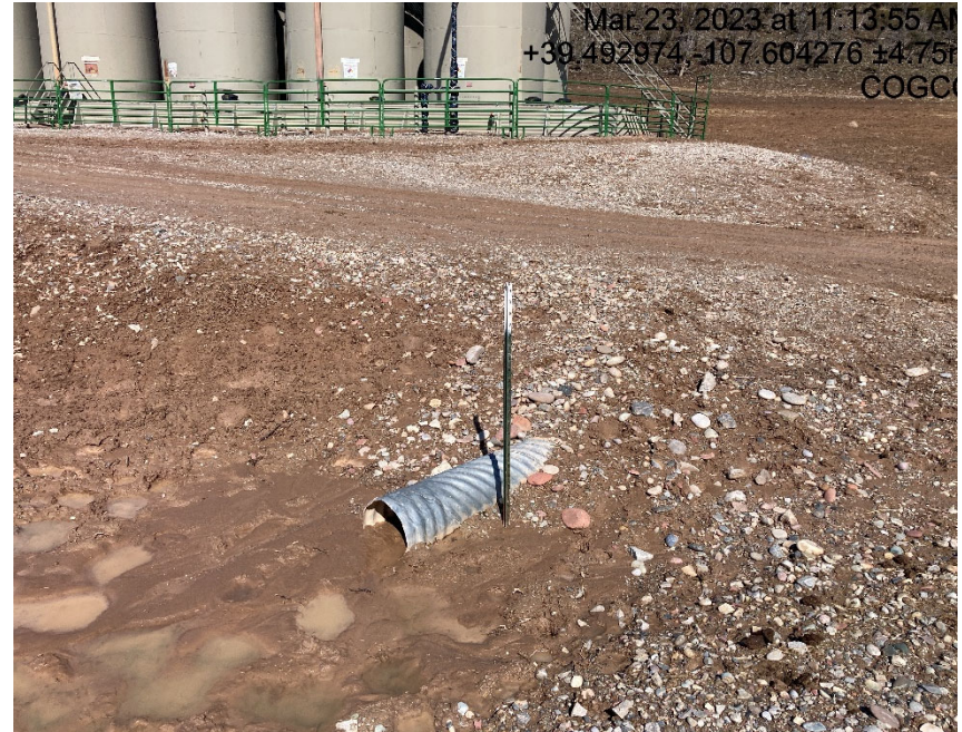
Culvert needs maintained
