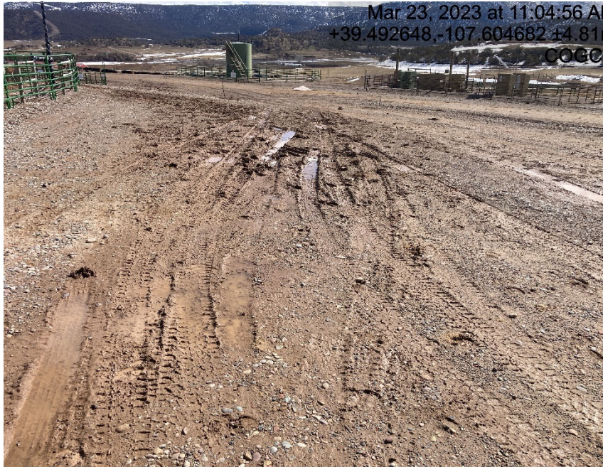
Lack of stabilization/compaction
