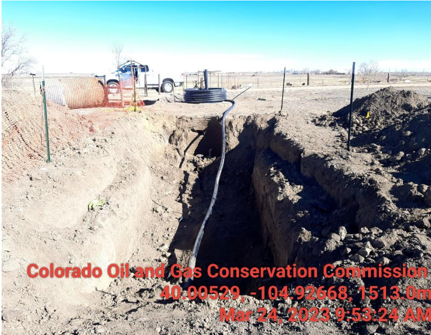
Photo 1 North end of line replacement operator installed a 3" SDR 11 line inside of a 4' steel line.
