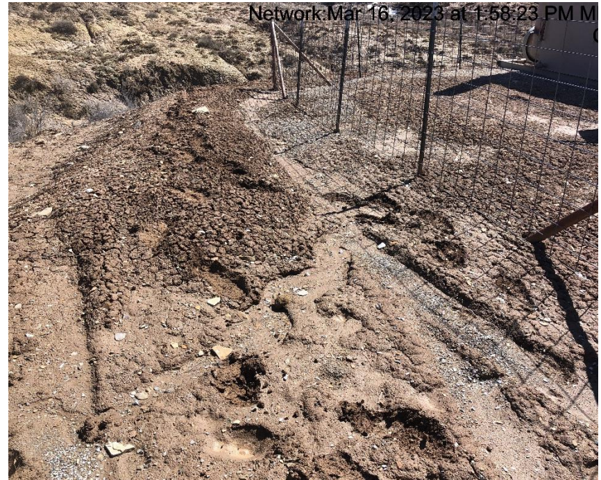
Photo #9358 Berms insufficient.
