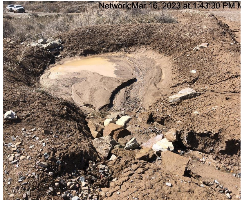
Photo #9368 Sediment traps insufficient.
