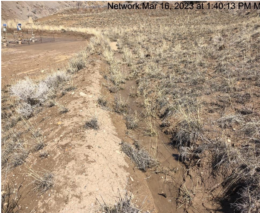
Photo #9316 Ditches insufficient.
