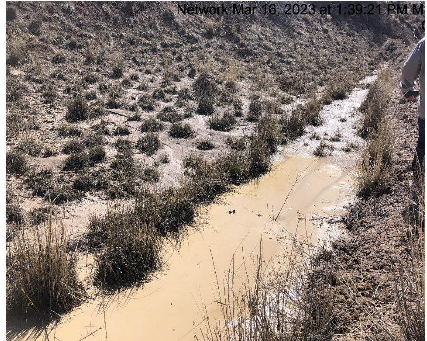
Photo #9312 Ditches insufficient.
