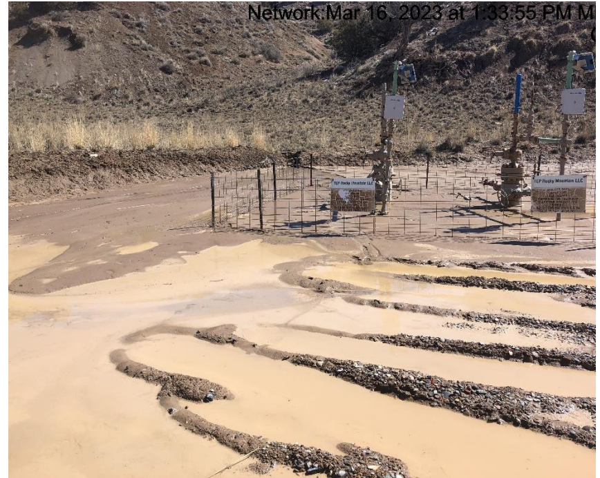
Photo #9294 Run on to location is not being controlled.
