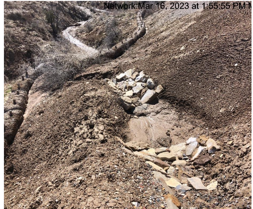
Photo #9354 Sediment trap insufficient
