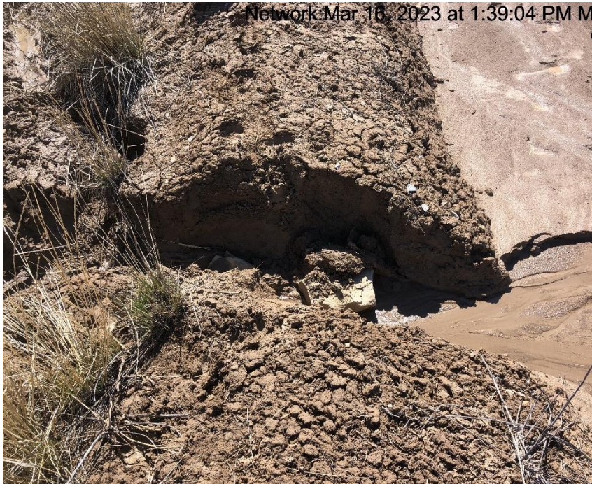
Photo #9310 Berms insufficient.
