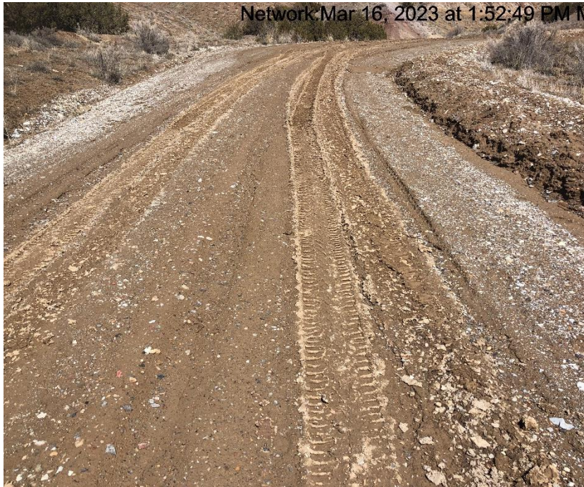
Photo #9345 Location lacks stabilization
