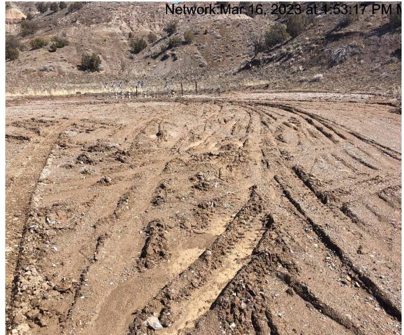
Photo #9347 Location lacks stabilization.
