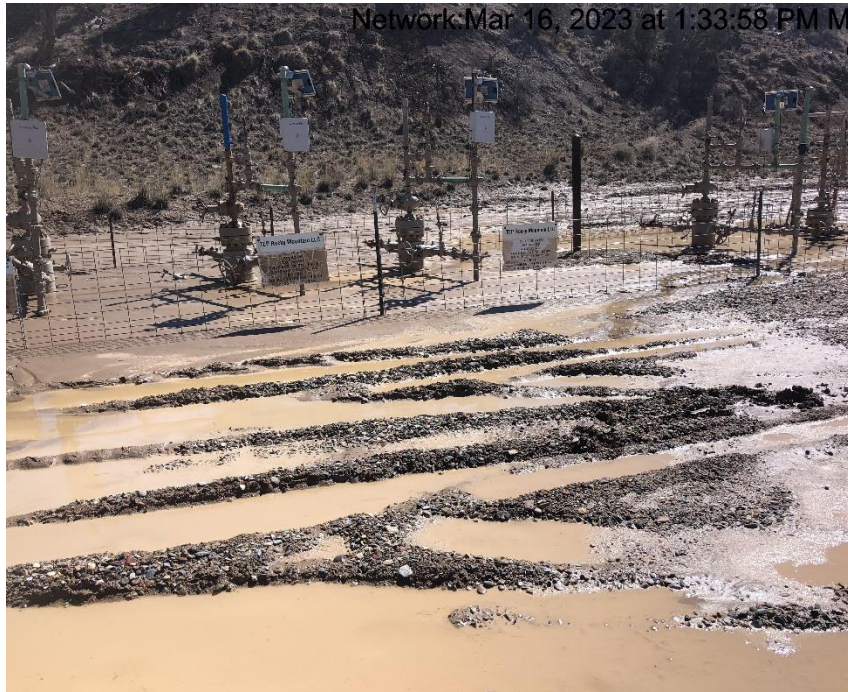
Photo #9295 Sediment encroaching on equipment.
