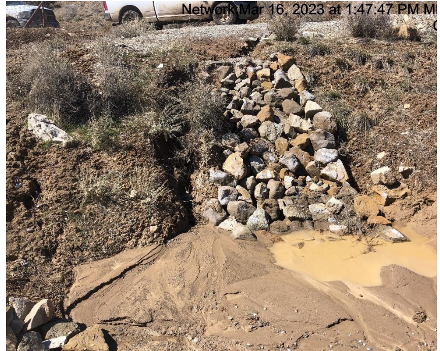
Photo #9340 Rip rap BMP insufficient
