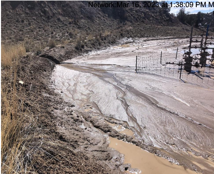
Photo #9338 Run on to location is not being controlled.
