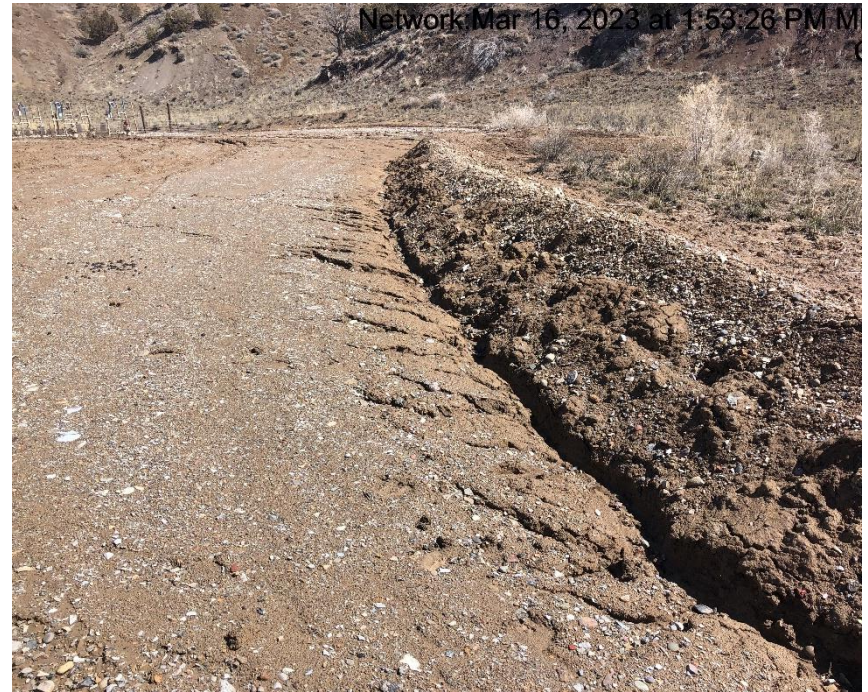
Photo #9349 Insufficient velocity BMPs.
