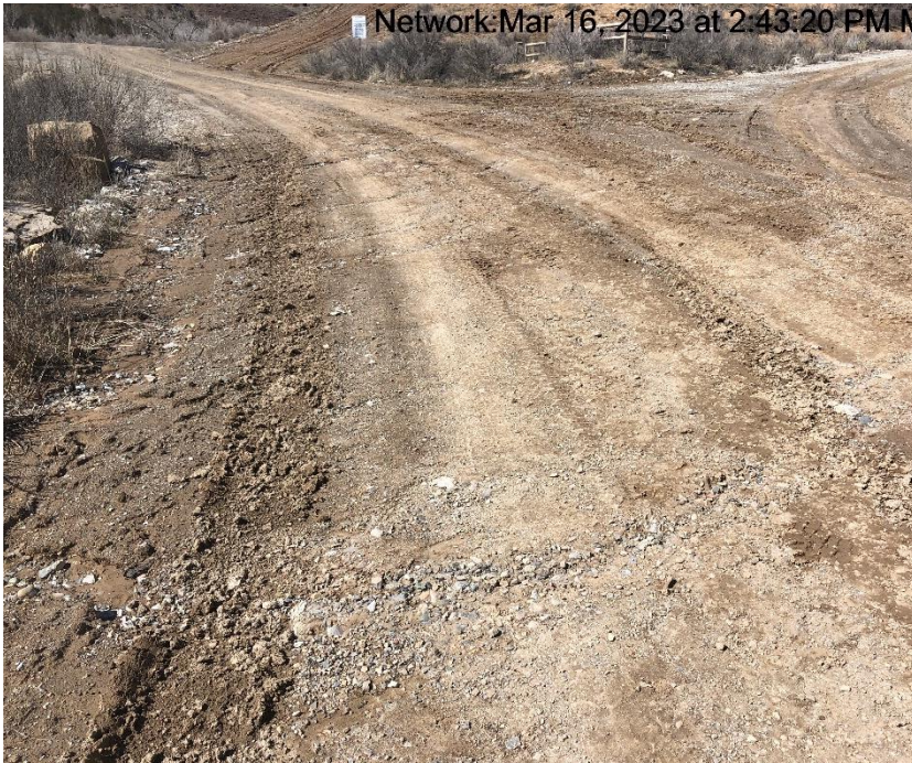
Photo #9368 Insufficient tracking BMP.
