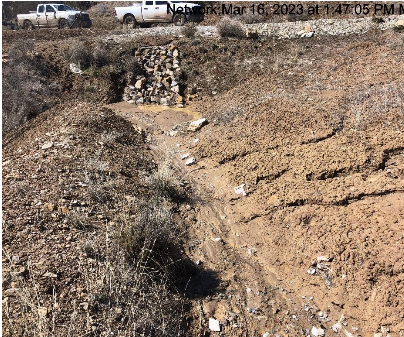
Photo #9338 Sediment trap insufficient
