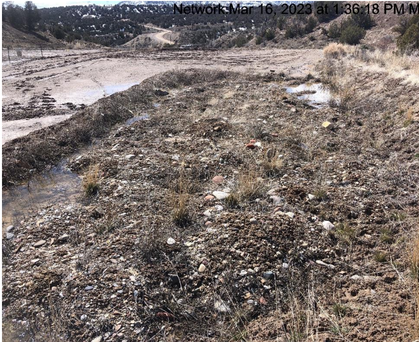
Photo #9301 Insufficient Stock piled soils BMPs.
