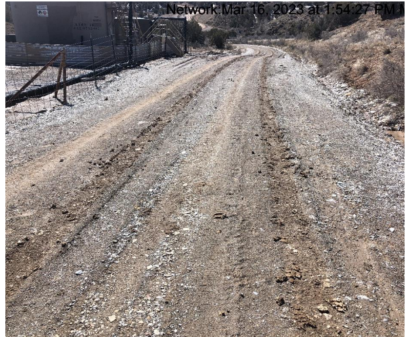
Photo #9353 Insufficient tracking BMP.
