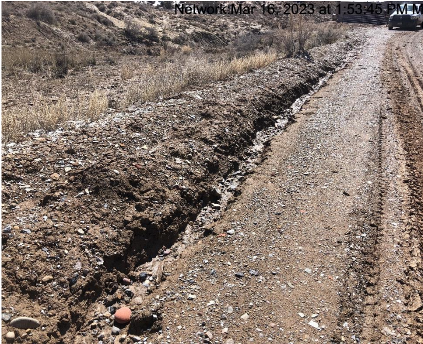
Photo #9351 Insufficient velocity BMPs.
