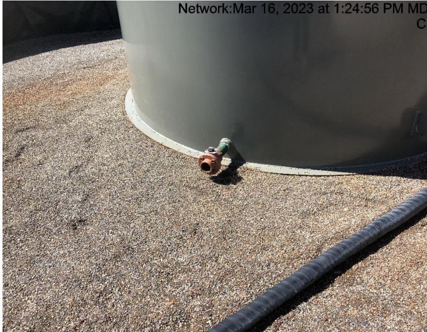
Photo #9286 Multiple loadlines open ended.
