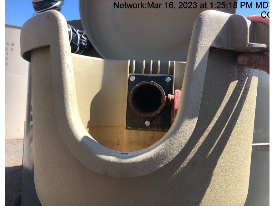
Photo #9287 Multiple loadlines open ended.
