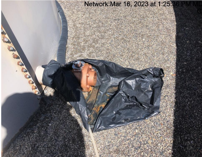
Photo #9288 Multiple loadlines open ended.
