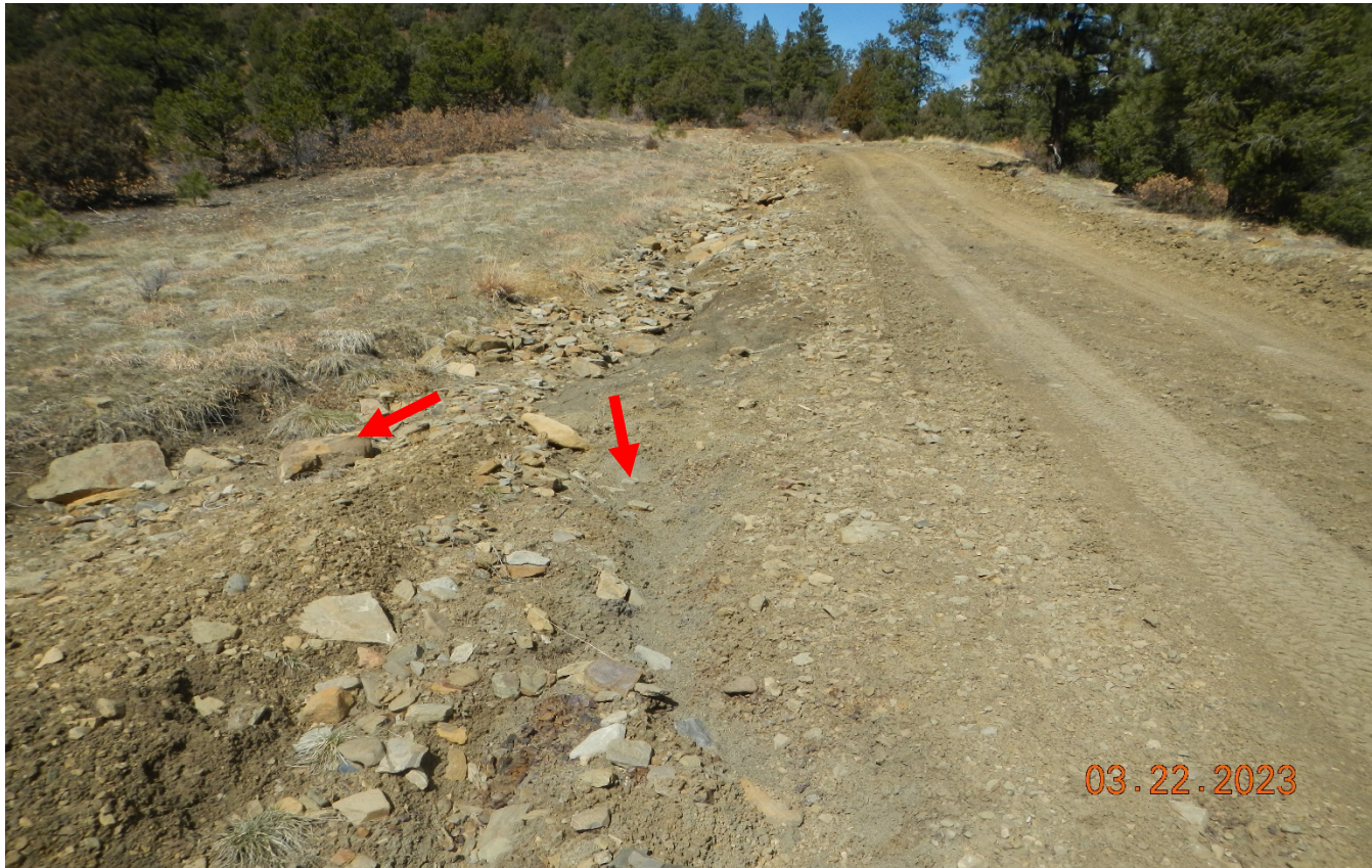
Photo 1. Facing northwest along the main road near the VPR C 140. Stormwater has caused erosion past the diversion which will continue to erode down the roadside.
