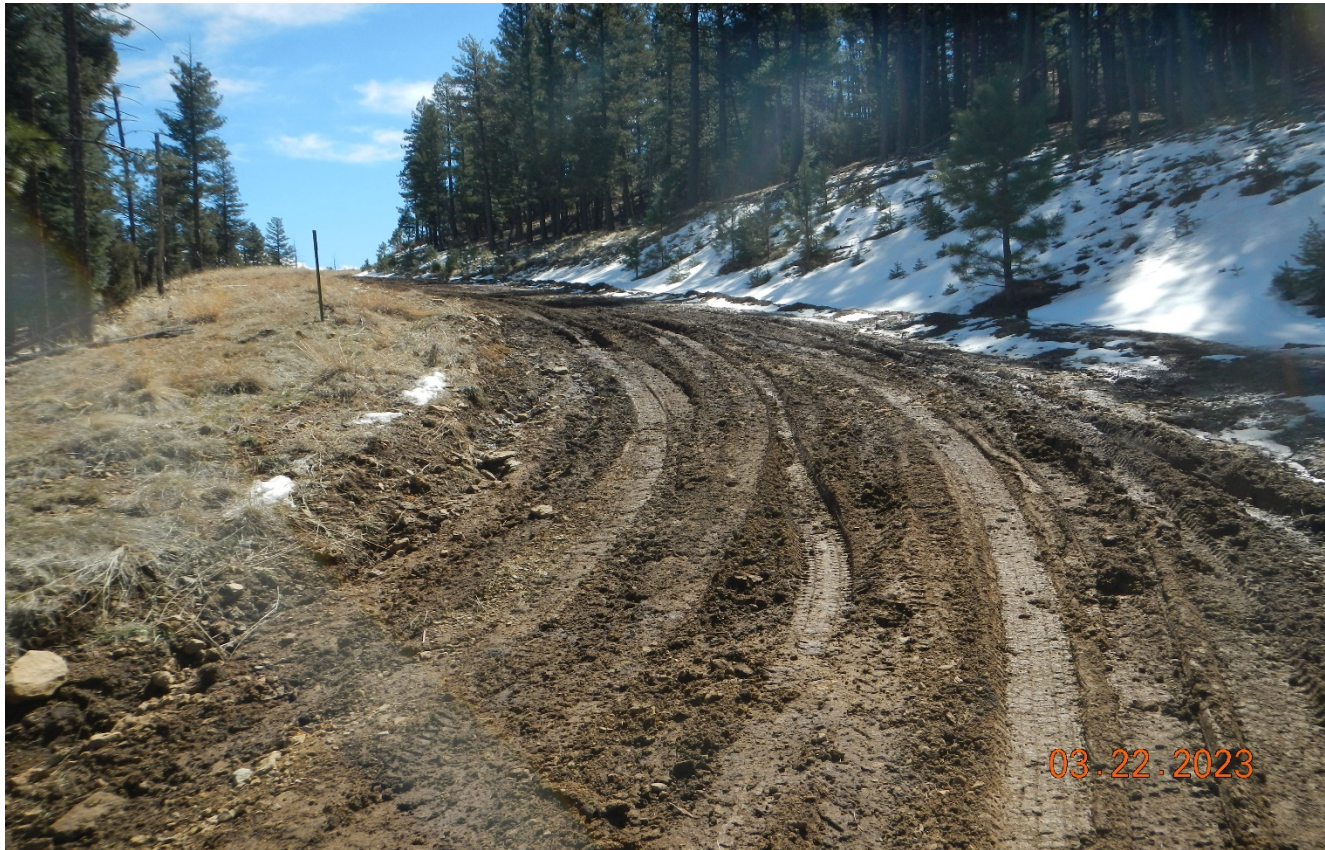
Photo 3. The road is rutted and not stabilized at the switch back of the main road traveling to the location.
