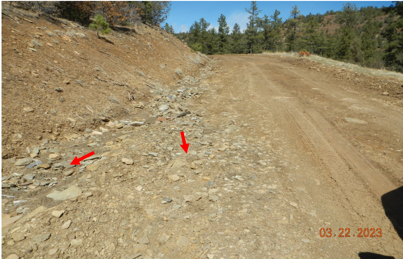
Photo 2. Facing northwest along the main road near the VPR C 140. Stormwater has caused erosion past the diversion which will continue to erode down the roadside.
