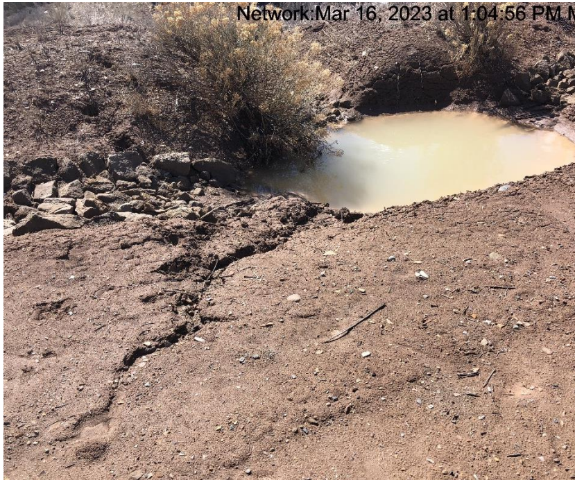
Photo #9273 Sediment trap in need of maintenance
