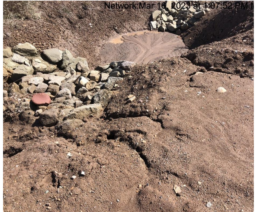
Photo #9281 Rill erosion into sediment trap.
