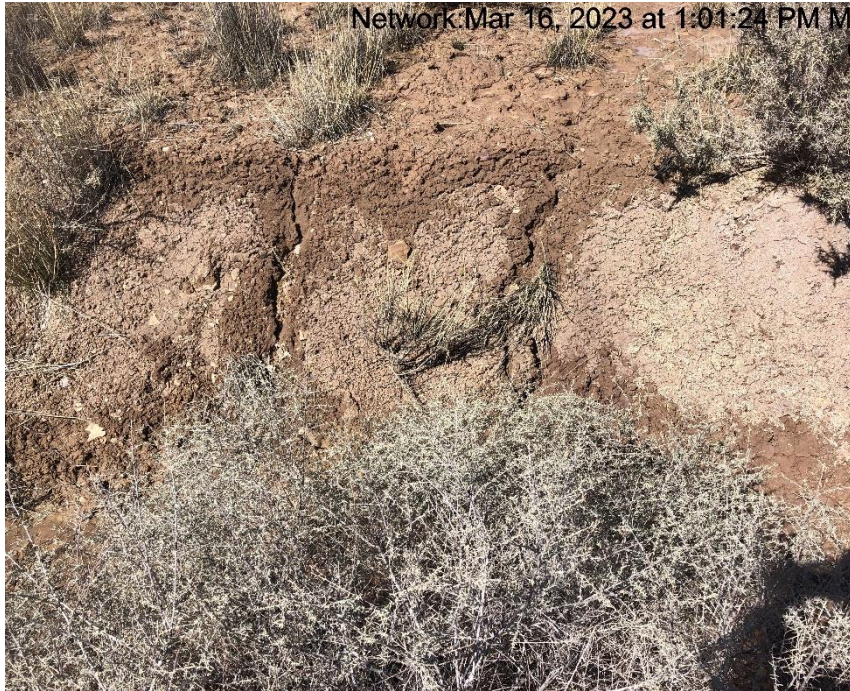
Photo #9267 Sediment trap and ditch degradation.
