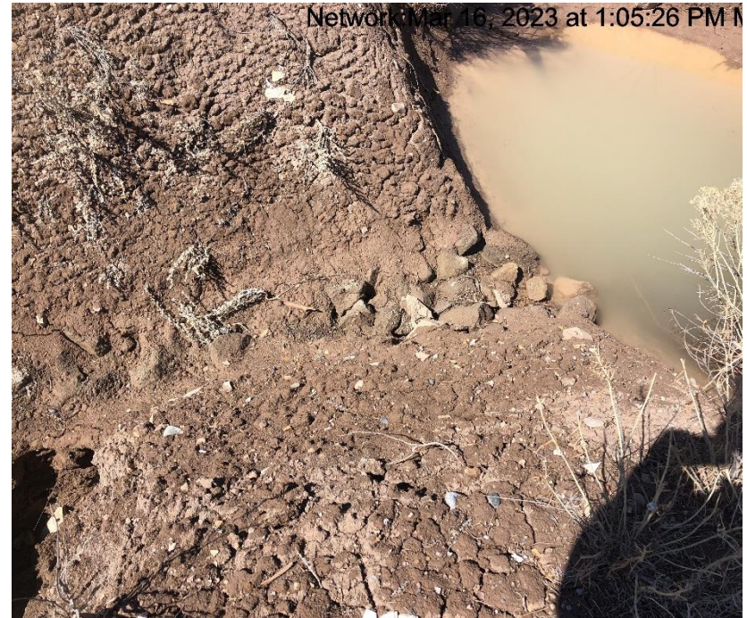
Photo #9274 Sediment trap in need of maintenance
