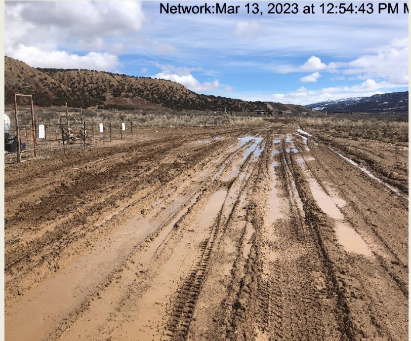
Photo #9246 Access road lacks stabilization.
