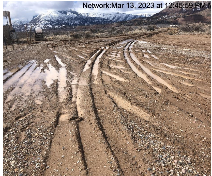
Photo #9237 Location lacks stabilization.
