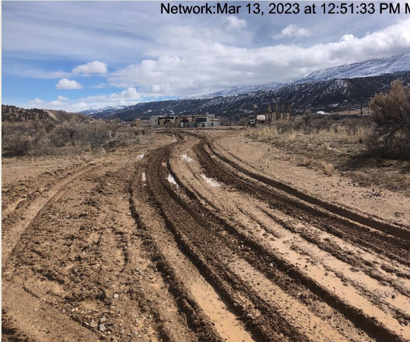
Photo #9245 Access road lacks stabilization.
