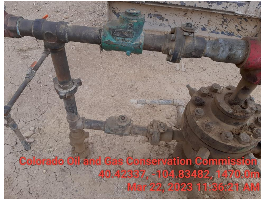
Photo 4 flow line appear to be in the open position on Genesis #3
