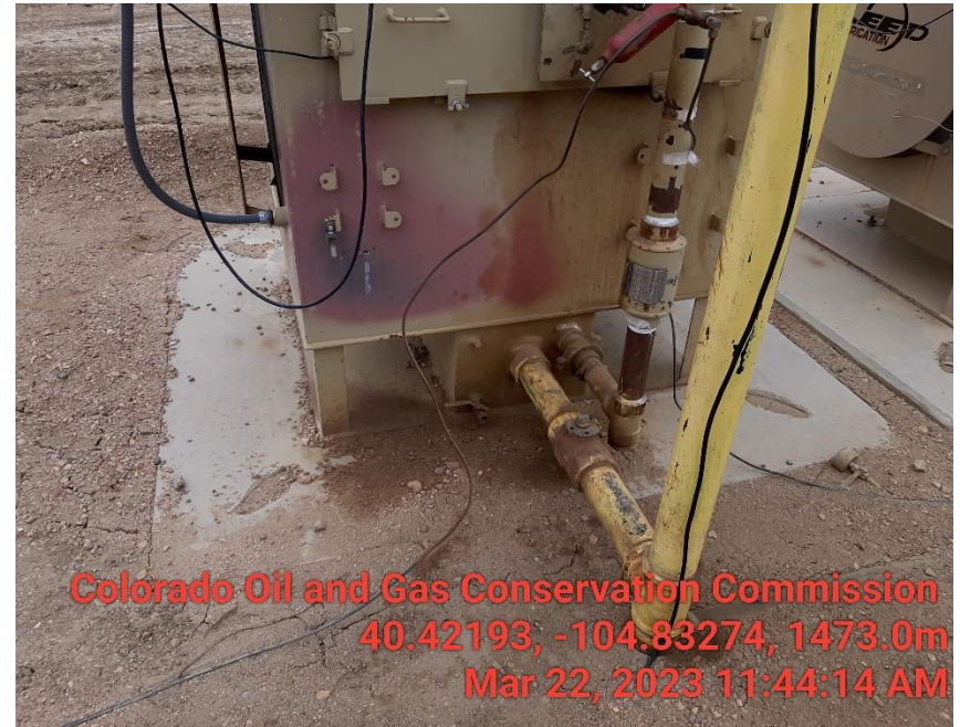
Photo 10 Stained soil/Mechanical issue piping on ECD
