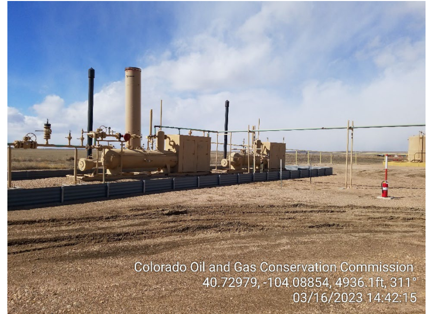
Photo 4 – Separators and ECD
