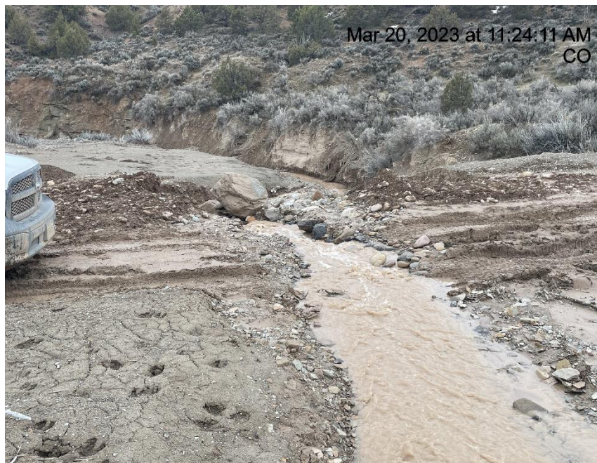
Photo # 2616 Degradation of roadway/insufficient BMP's
