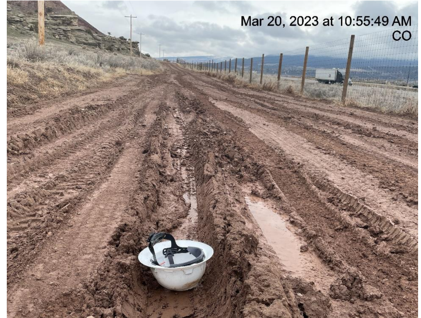
Photo # 2602 Lack of stabilization on lease road
