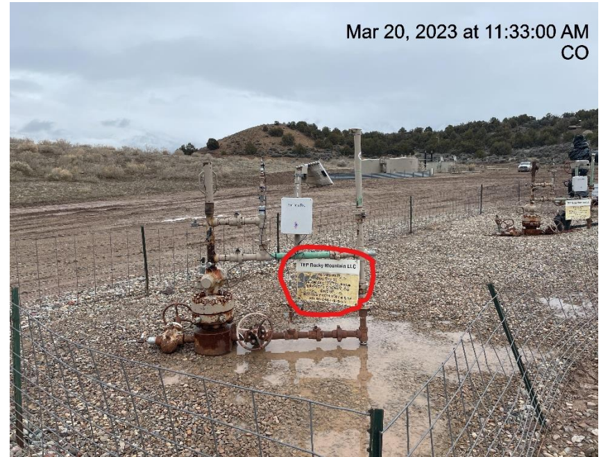
Photo # 2626 Wellhead sign peeling & illegible
