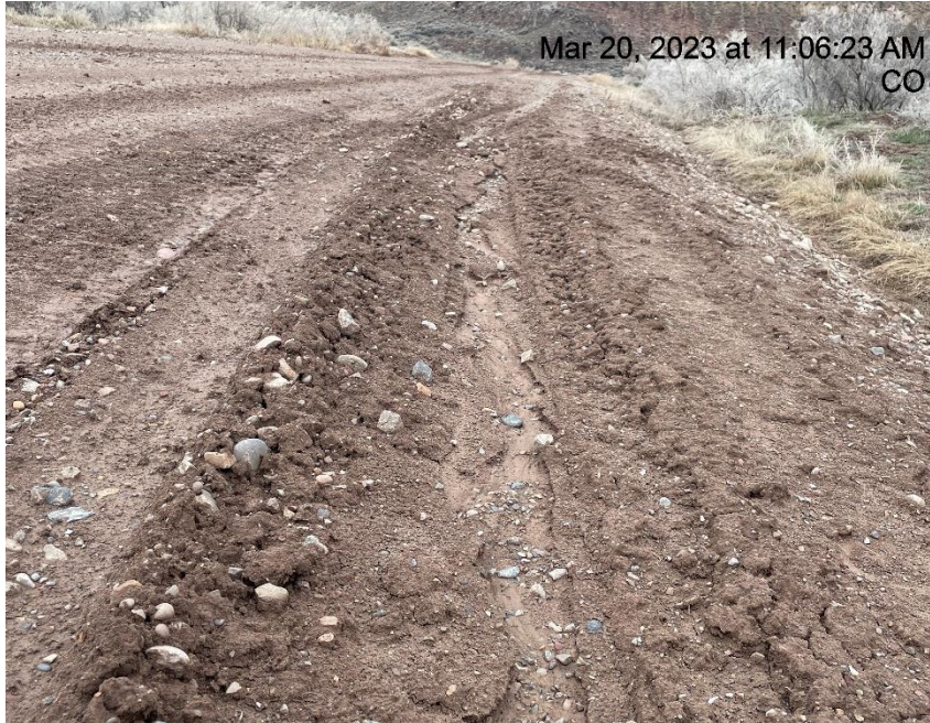
Photo # 2608 Rill erosion on lease road
