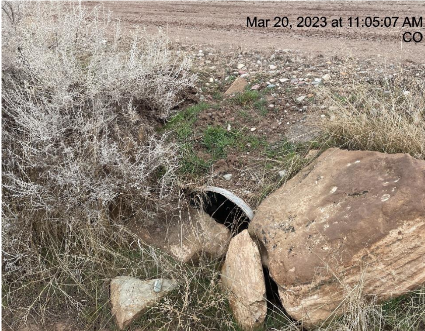
Photo # 2606 Culvert needs maintenance
