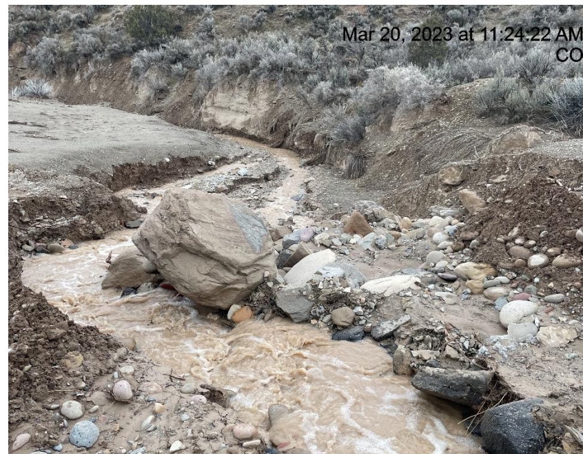
Photo # 2617 Degradation of roadway/insufficient BMP's
