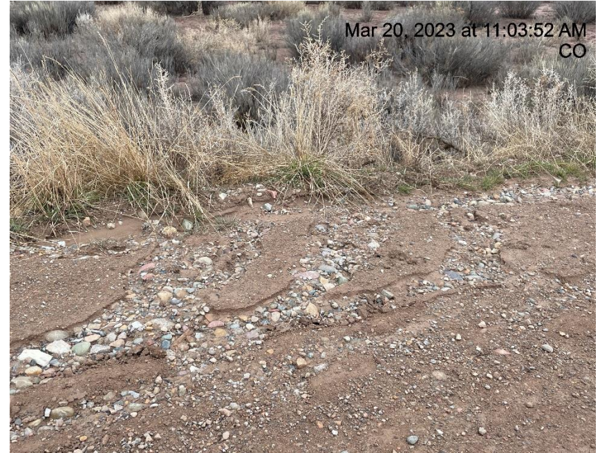
Photo # 2605 Rill erosion on lease road
