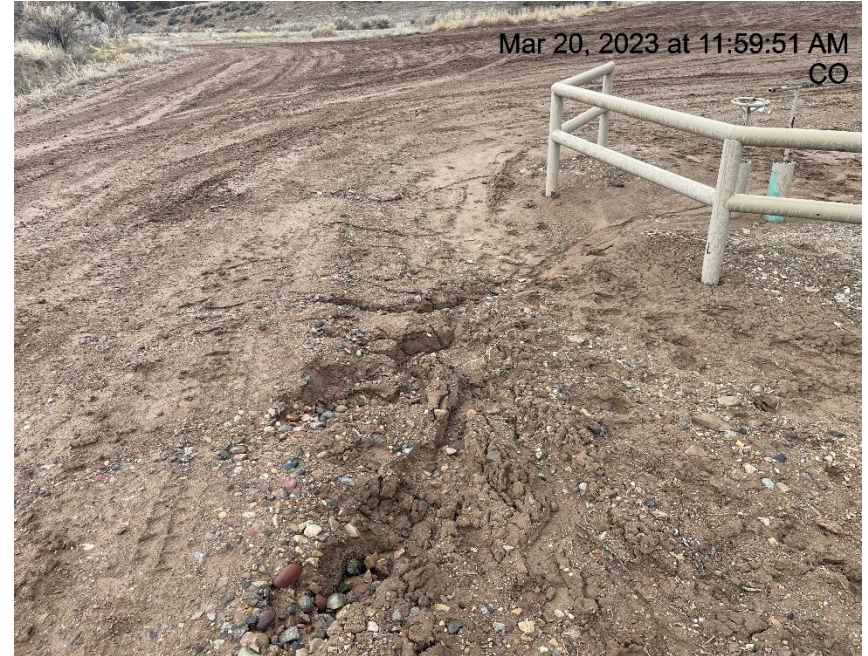
Photo # 2651 Gully erosion near bollards at entrance to location
