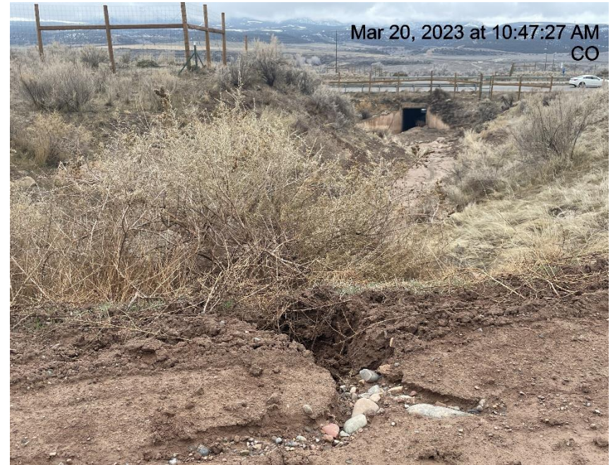
Photo # 2595 Gully erosion
