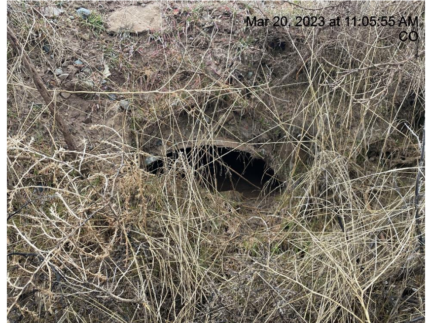
Photo # 2607 Culvert needs maintenance
