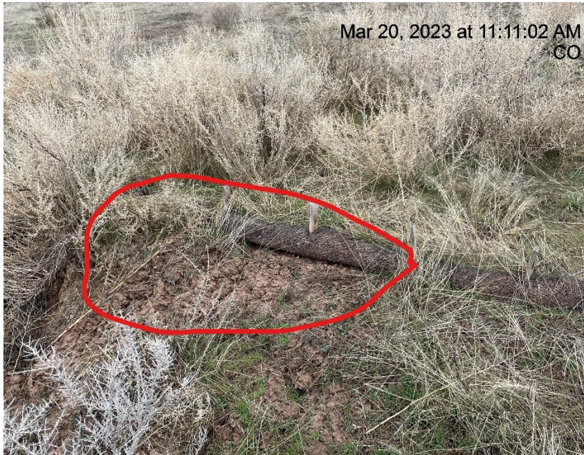
Photo # 2609 Waddles around culvert need maintenance
