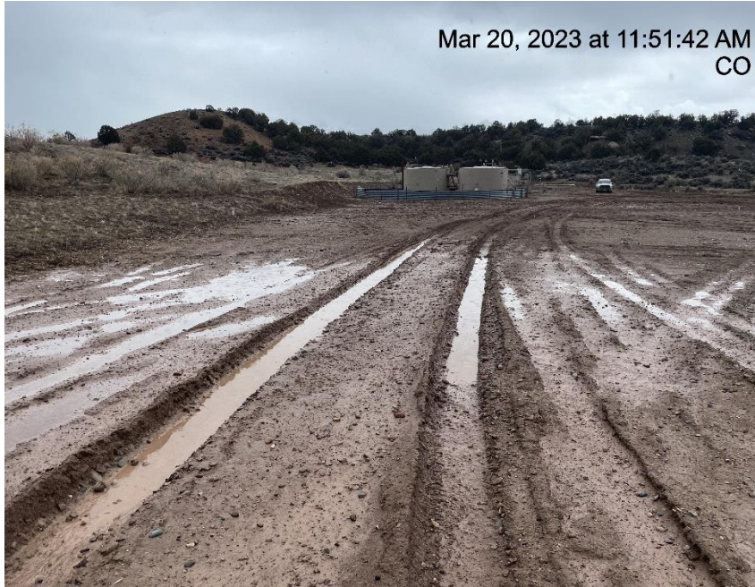
Photo # 2643 Lack of stabilization
