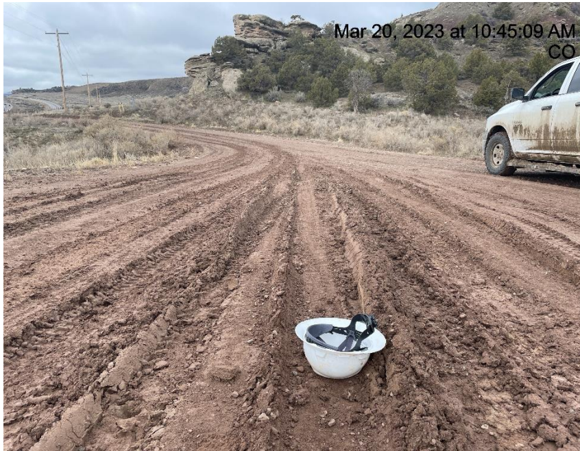
Photo # 2593 Lack of stabilization on lease road
