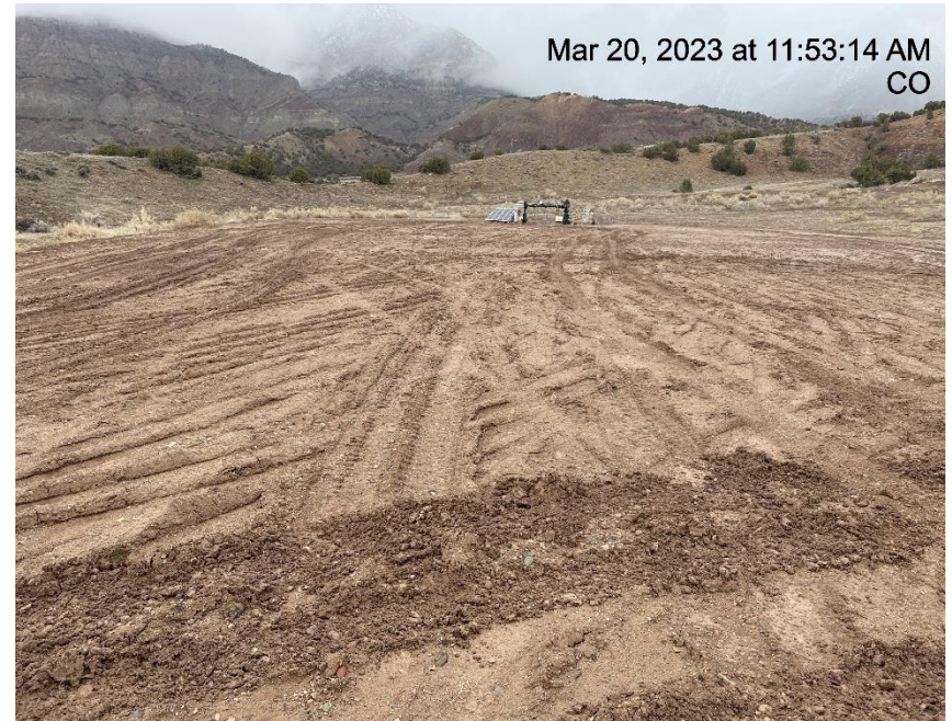
Photo # 2645 Lack of stabilization
