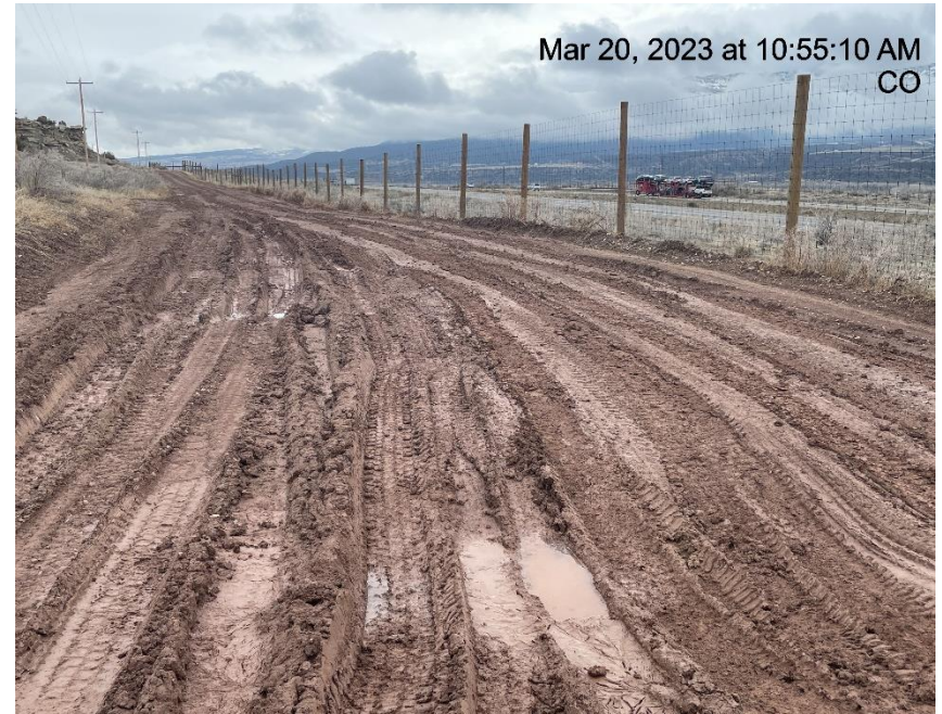
Photo # 2599 Lack of stabilization on lease road
