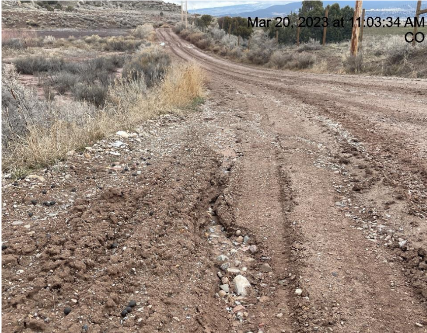
Photo # 2603 Rill erosion on lease road
