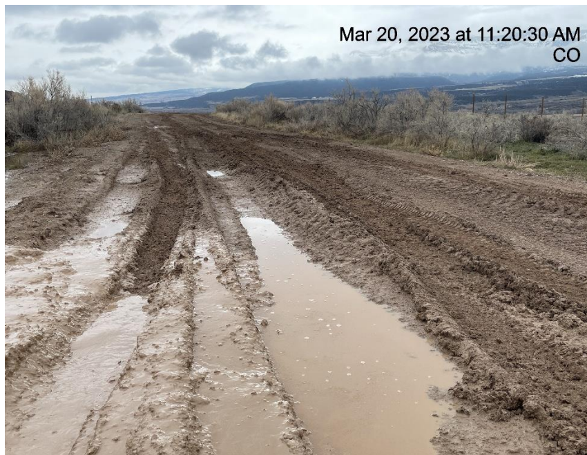
Photo # 2612 Lack of stabilization on lease road
