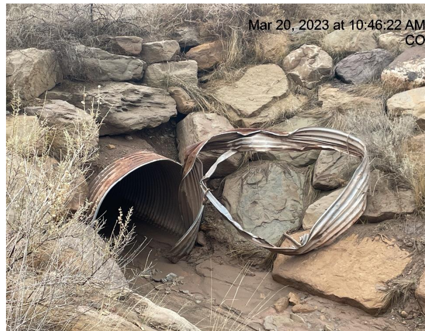
Photo # 2594 Culvert needs maintenance
