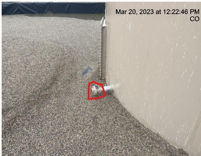
Photo # 2680 Open ended load line
