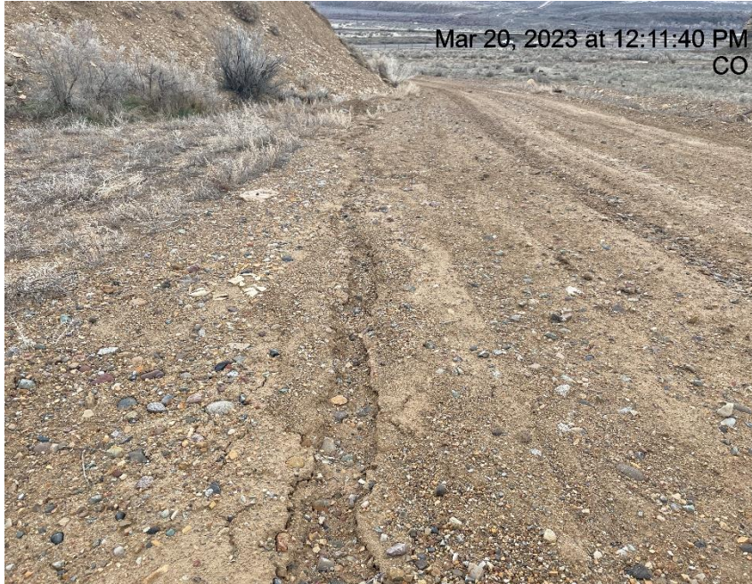
Photo # 2665 Rill erosion on spur road
