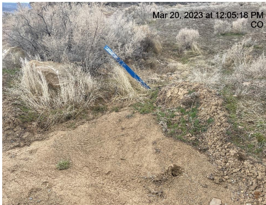
Photo # 2660 Erosion & Transport of sediment off spur road
