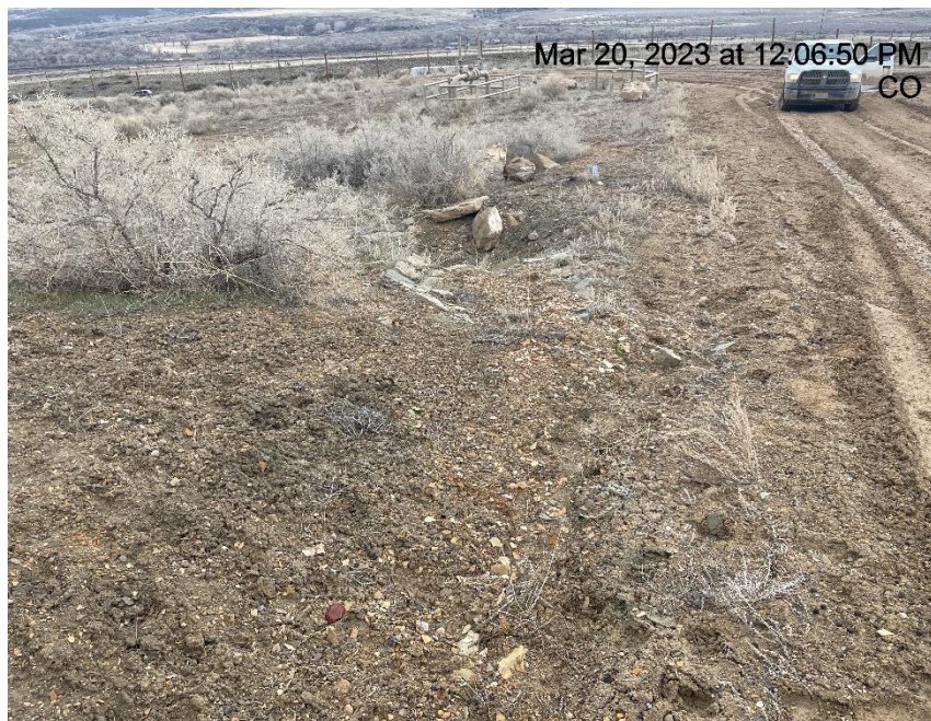
Photo # 2664 Sediment trap & ditch need maintenance
