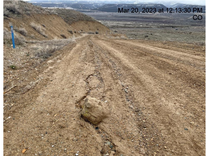
Photo # 2667 Rill erosion on spur road
