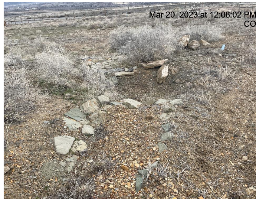
Photo # 2662 Sediment trap needs maintenance
