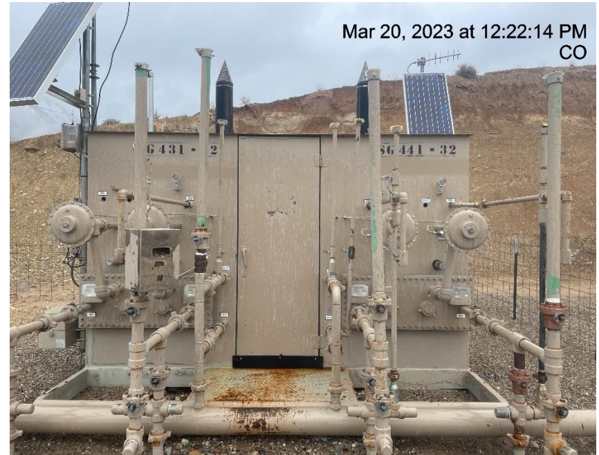
Photo # 2679 Meter calibration info not conspicuously posted
