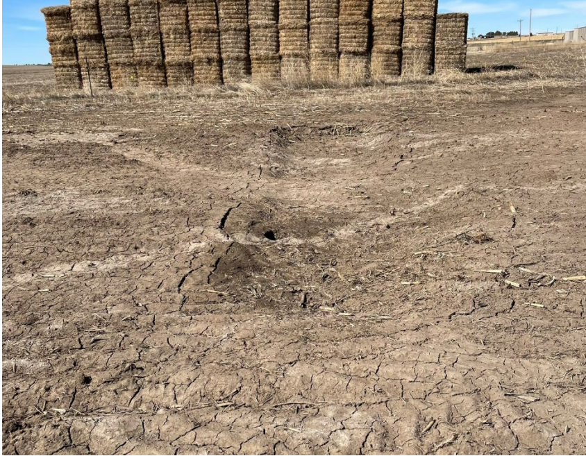
Photo 3 – Subsidence around former tank battery
