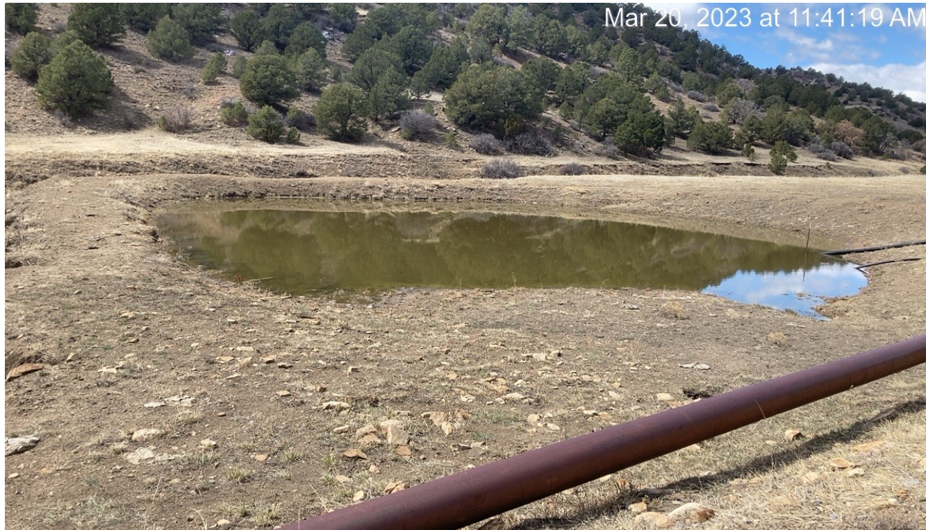
Photo 1. The water in the pit is above 2 ft. freeboard. Notified Evergreen employee that was at the location.
