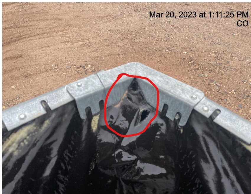
Photo # 2718 Containment liner needs maintenance
