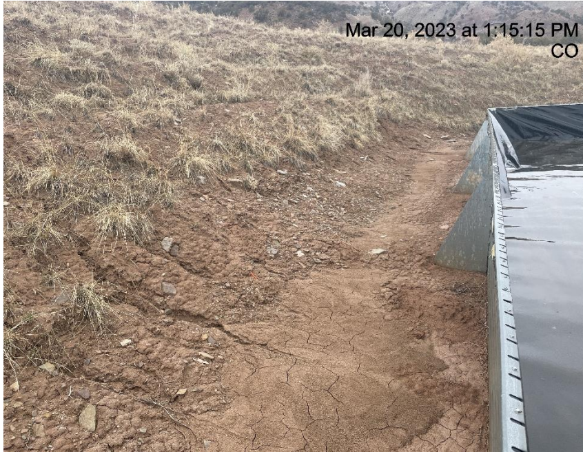
Photo # 2723 Rill erosion/insufficient run on control (BMP)/sediment encroaching on equipment
