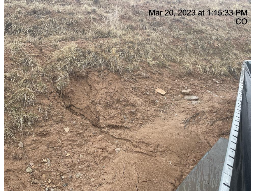
Photo # 2724 Rill erosion/insufficient run on control (BMP)/sediment encroaching on equipment
