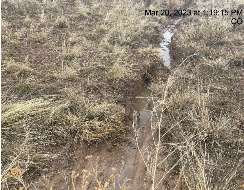
Photo # 2726 Channel erosion/insufficient BMP
