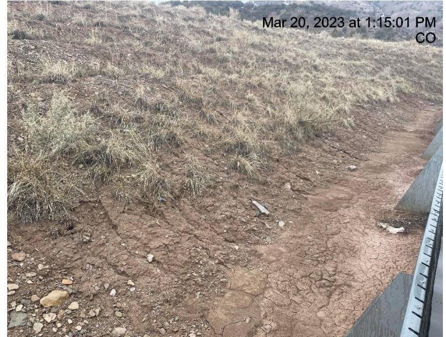
Photo # 2722 Rill erosion/insufficient run on control (BMP)/sediment encroaching on equipment
