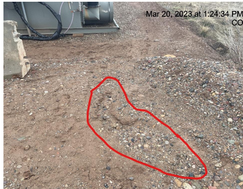
Photo # 2738 Gulley erosion near entrance to location
