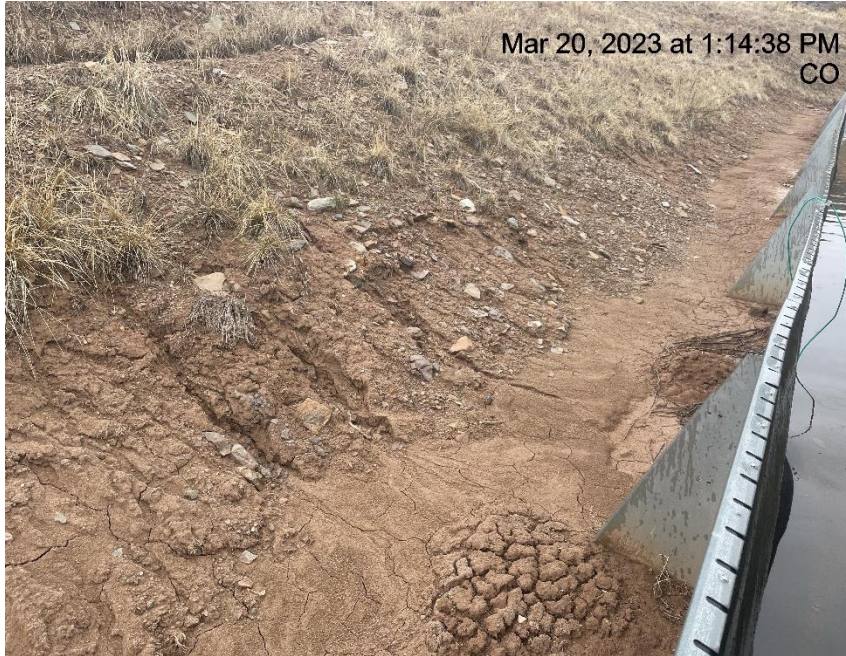
Photo # 2720 Rill erosion/insufficient run on control (BMP)/sediment encroaching on equipment
