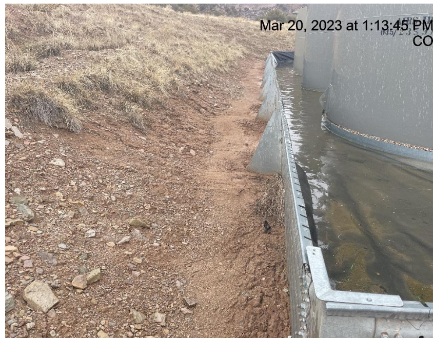
Photo # 2719 Rill erosion/insufficient run on control (BMP)/sediment encroaching on equipment
