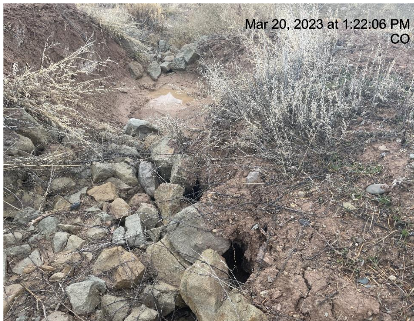
Photo # 2733 Sediment Trap needs maintenance
