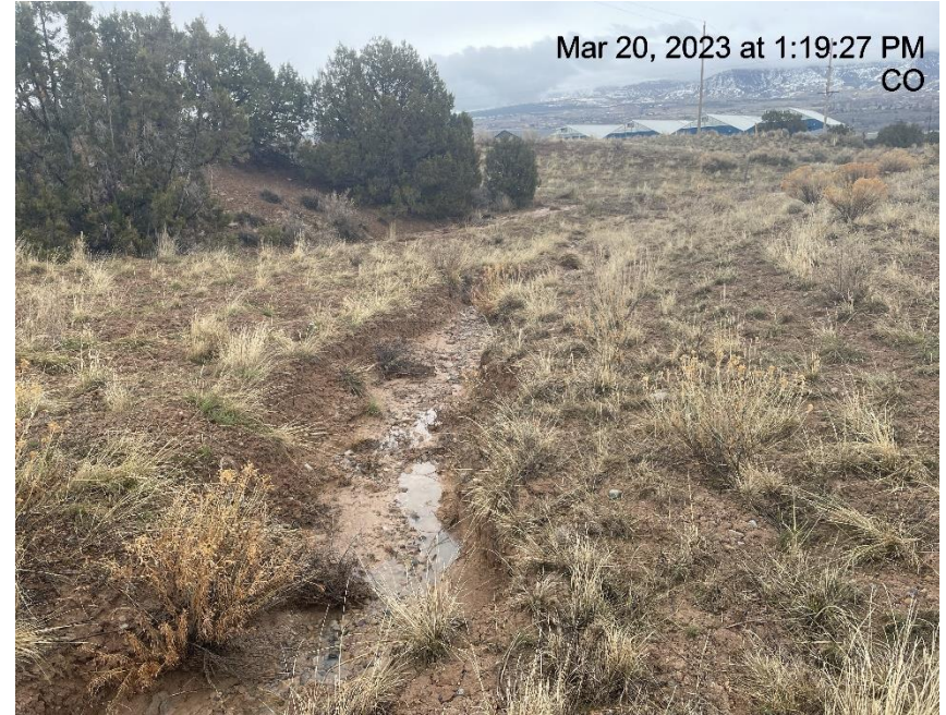
Photo # 2727 Channel erosion/insufficient BMP
