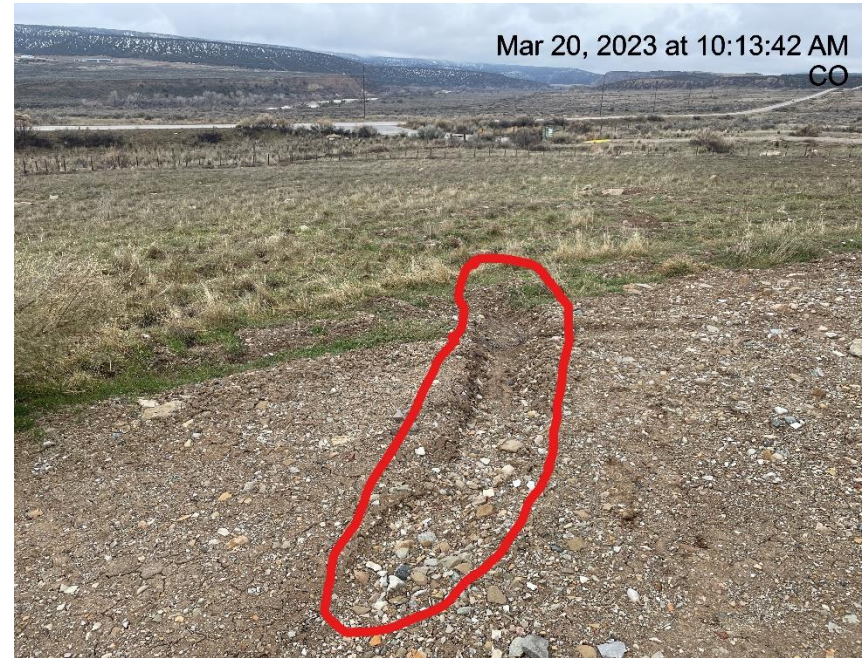
Photo # 2584 Gulley erosion on location, 40 yards SW of solar panels
