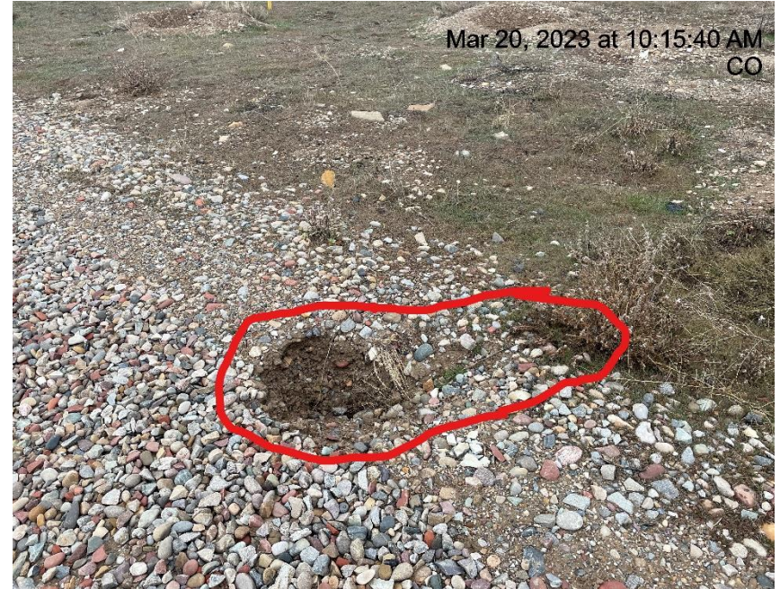
Photo # 2586 Gulley erosion on lease road 40 yards from tracking pad on the west side
