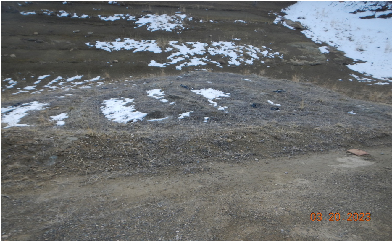
Photo 4. Facing toward the southeast side of the location. There is grey colored dirt piled up with remnants of pit liner debris. It appears the pit was excavated and material and liner was left in this area. The berm around the pit material is degraded and has not contained the material.
