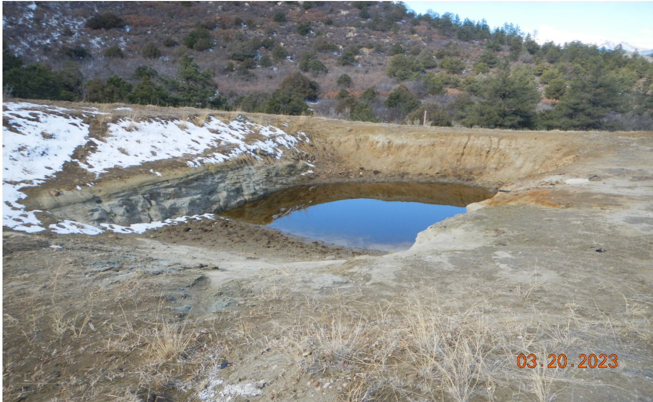
Photo 3. Facing toward the pit. Pit was permitted with liner however there is no liner in the pit. No freeboard marker.
