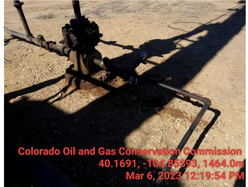
Photo 4 Stained soil and mechanical issue 1" Flow line
