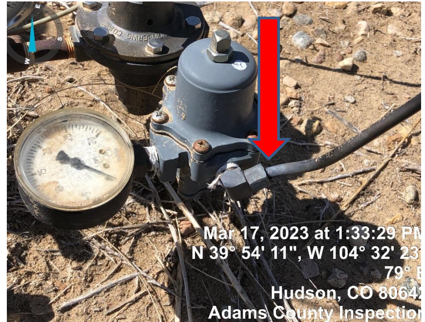
Photo#4 Fitting Leaking Gas
