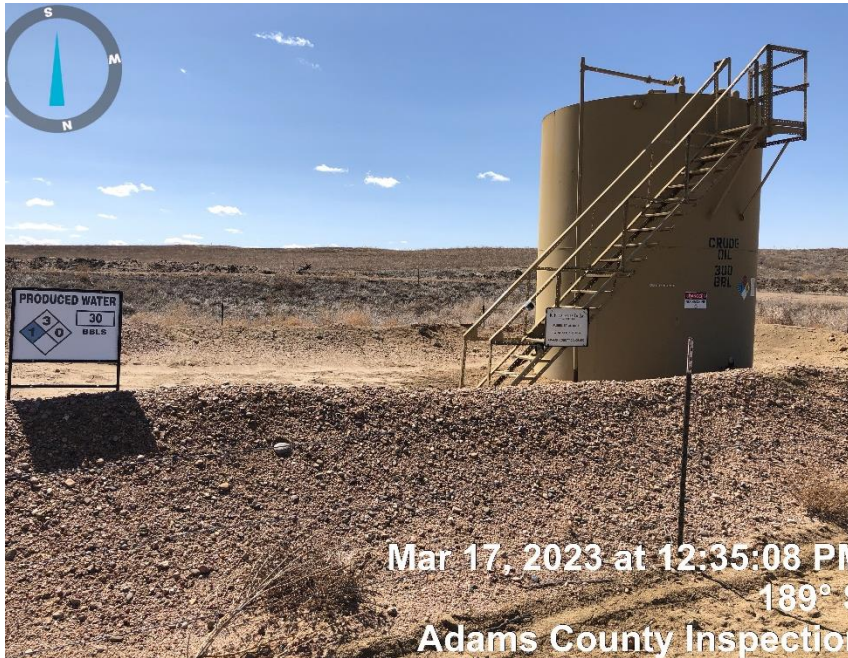
Photo#1 Production Tank and Produced Water Vault
