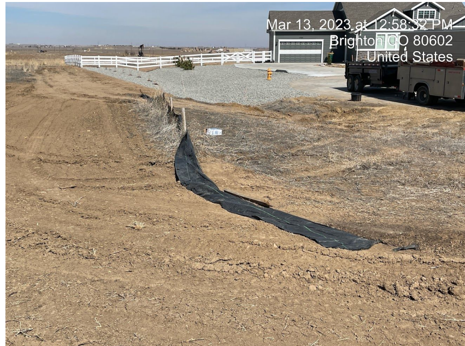
Photo 9. Photo of downed silt fence at entrance of location.
