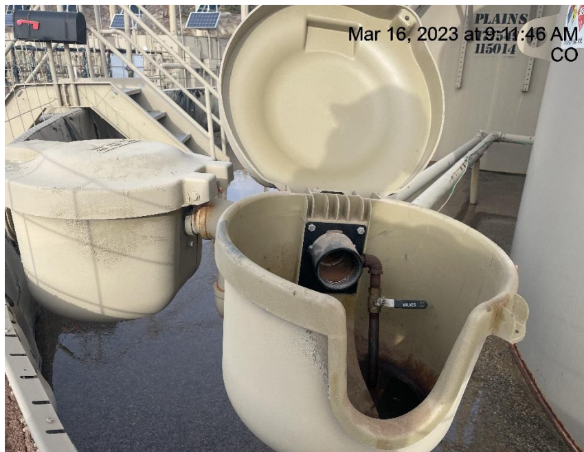
Photo # 2424 Open ended load line
