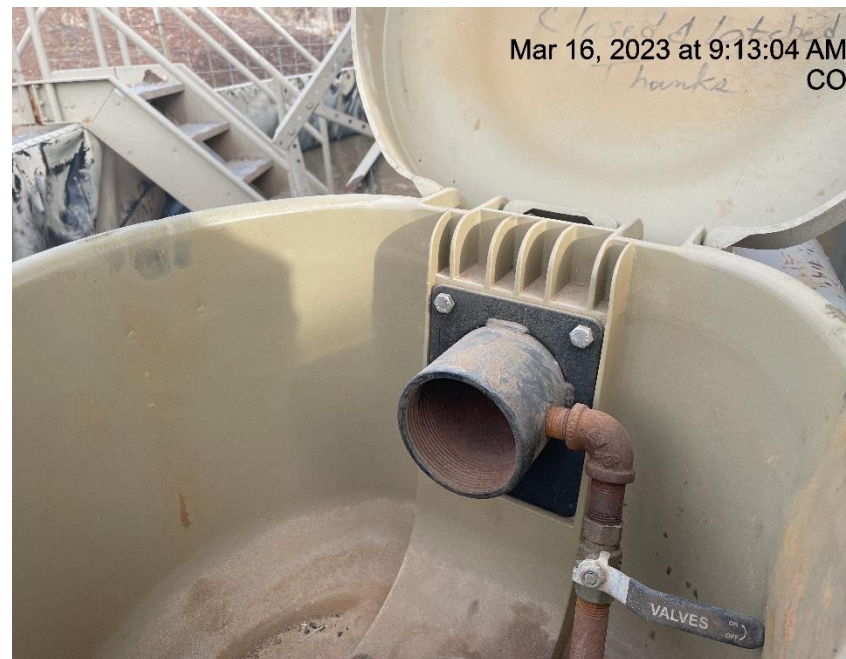
Photo # 2427 Open ended load line
