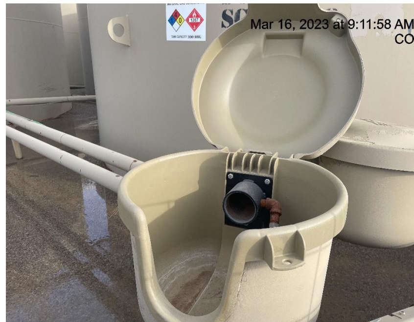
Photo # 2425 Open ended load line
