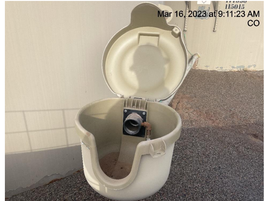
Photo # 2423 Open ended load line
