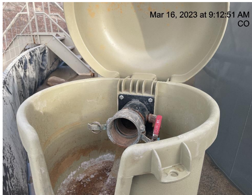
Photo # 2426 Open ended load line
