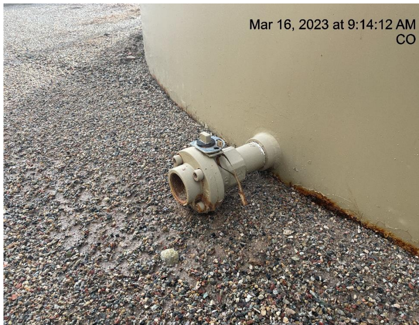
Photo # 2430 Open ended load line
