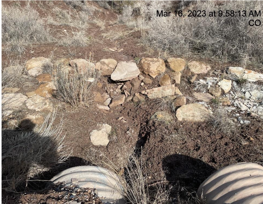
Photo # 2447 Rip Rap needs maintenance (on lease road approximately 600 yards past the I-70 underpass)
