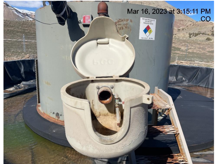
Photo # 2519 Open ended load line
