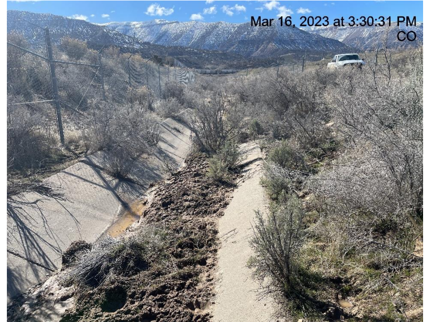
Photo # 2535 Ditch along lease road needs maintenance
