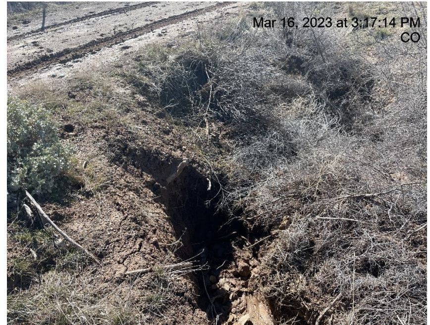
Photo # 2524 Culvert needs maintenance (lease road)
