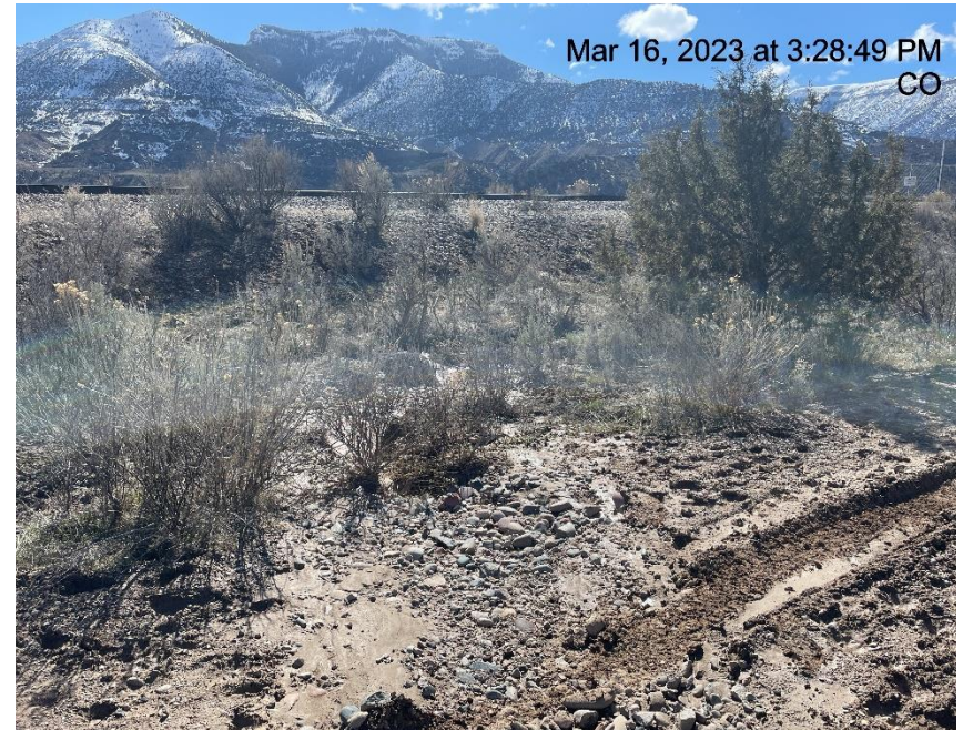
Photo # 2531 Erosion & sediment migration off lease road
