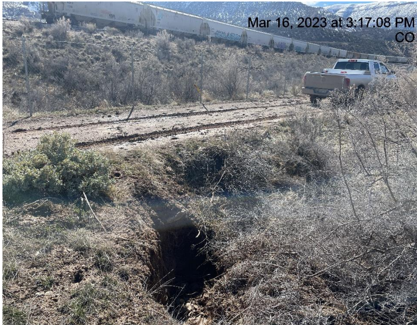
Photo # 2523 Culvert needs maintenance (lease road)
