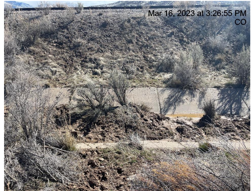
Photo # 2527 Ditch along lease road needs maintenance
