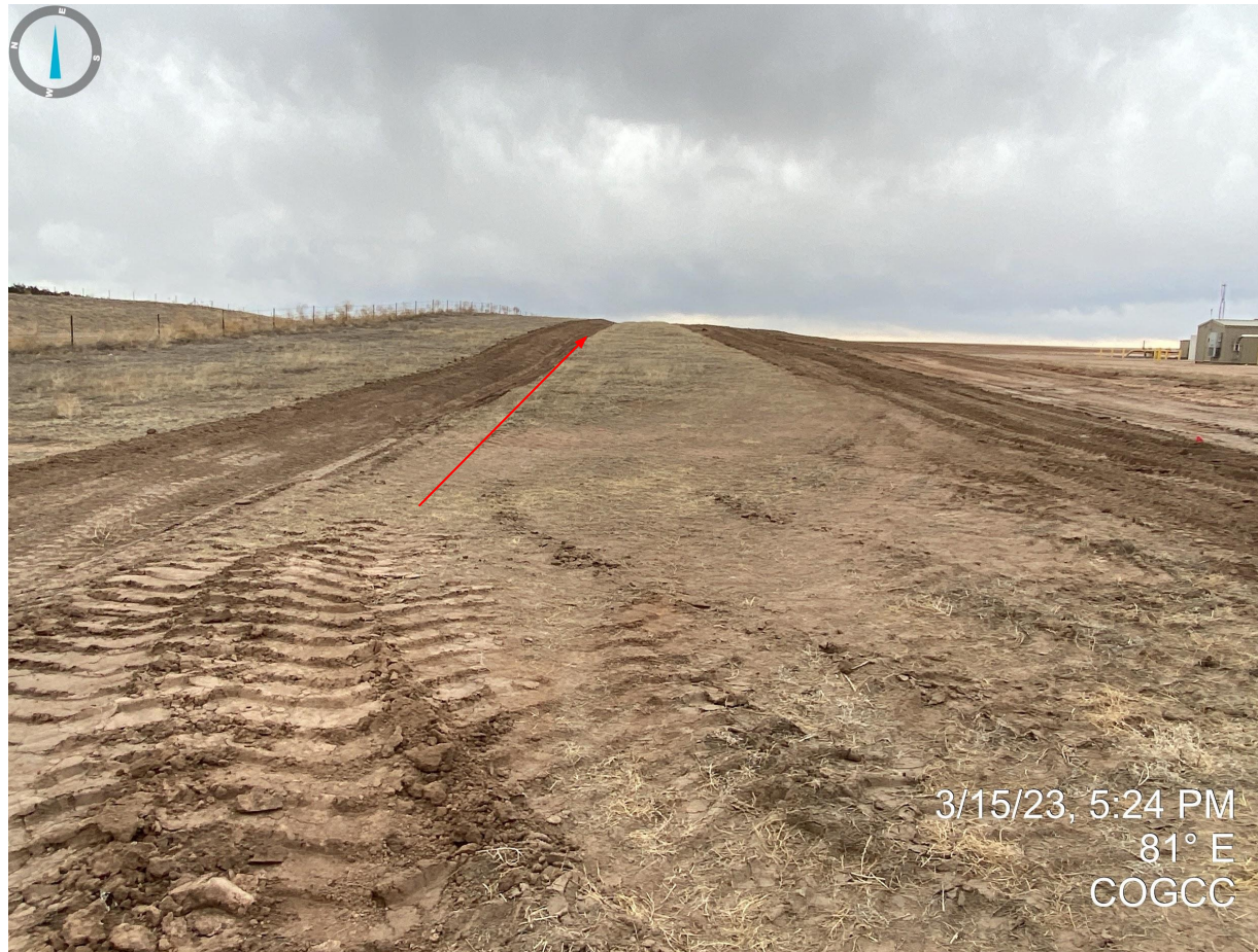
Photo 1. Facing east from the location entrance. Temporary BMPs have been installed (ditch and berm) around the entire perimeter during the construction phase of the location. More permanent BMPs should be installed upon the completion of pad expansion.
