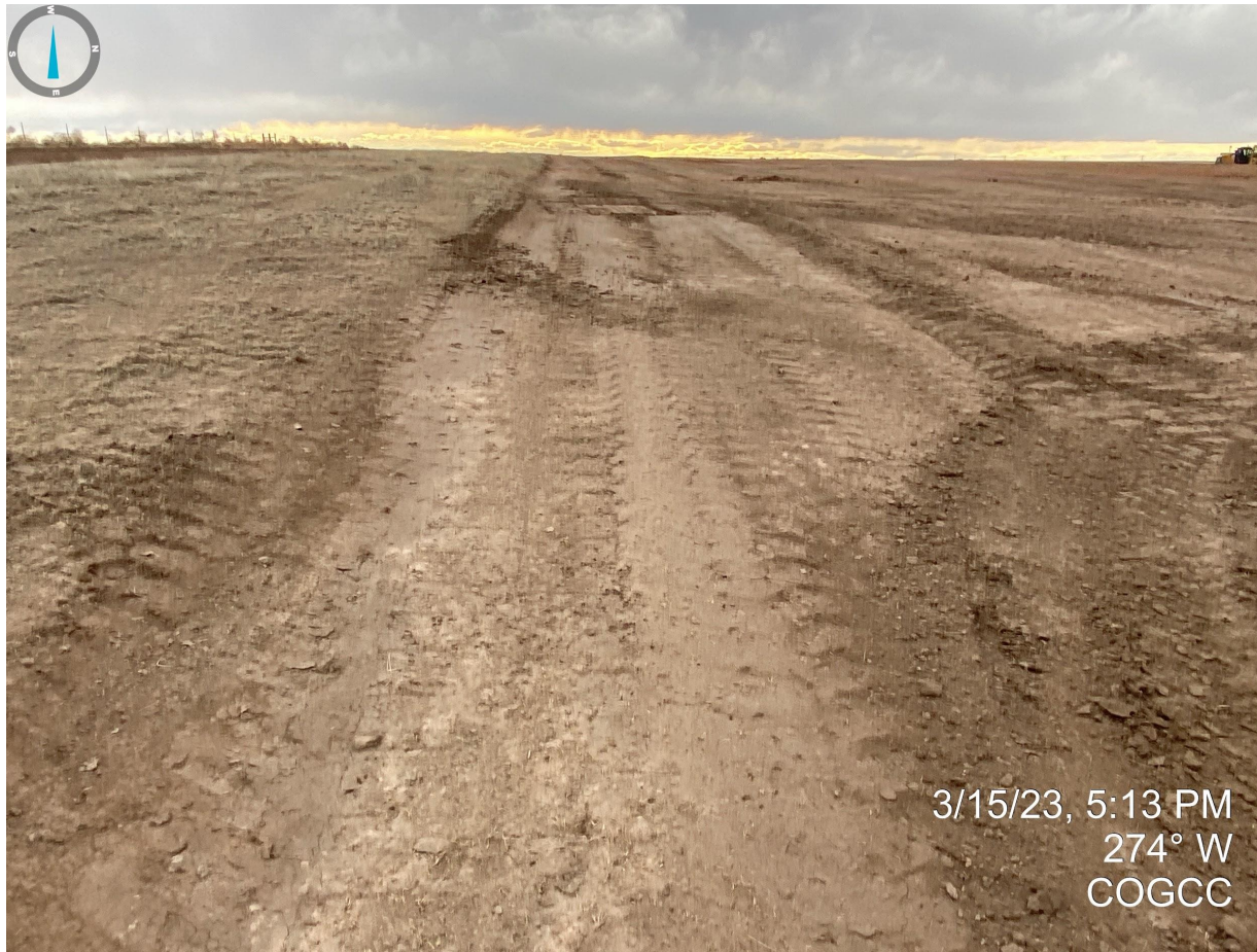
Photo 11. Facing west from the southern portion of the location. Topsoil salvage operations were still occurring during this inspection. The Operator shall ensure that all topsoil is properly salvaged and segregated.
