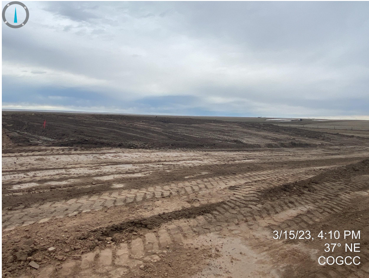
Photo 7. Facing northeast towards the new topsoil stockpile. Construction activities were occurring at the time of this inspection; topsoil salvage operations are still ongoing and the material is being segregated on the northeastern portion of the location.
