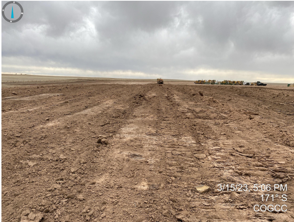
Photo 9. Facing south from topsoil stockpile; salvage operations were still on-going. Staff observed some evidence of equipment tracking on the stockpile and it is required by Rule 1002.c that the entire topsoil stockpile is temporarily stabilized prior to long term stabilization efforts occur.
