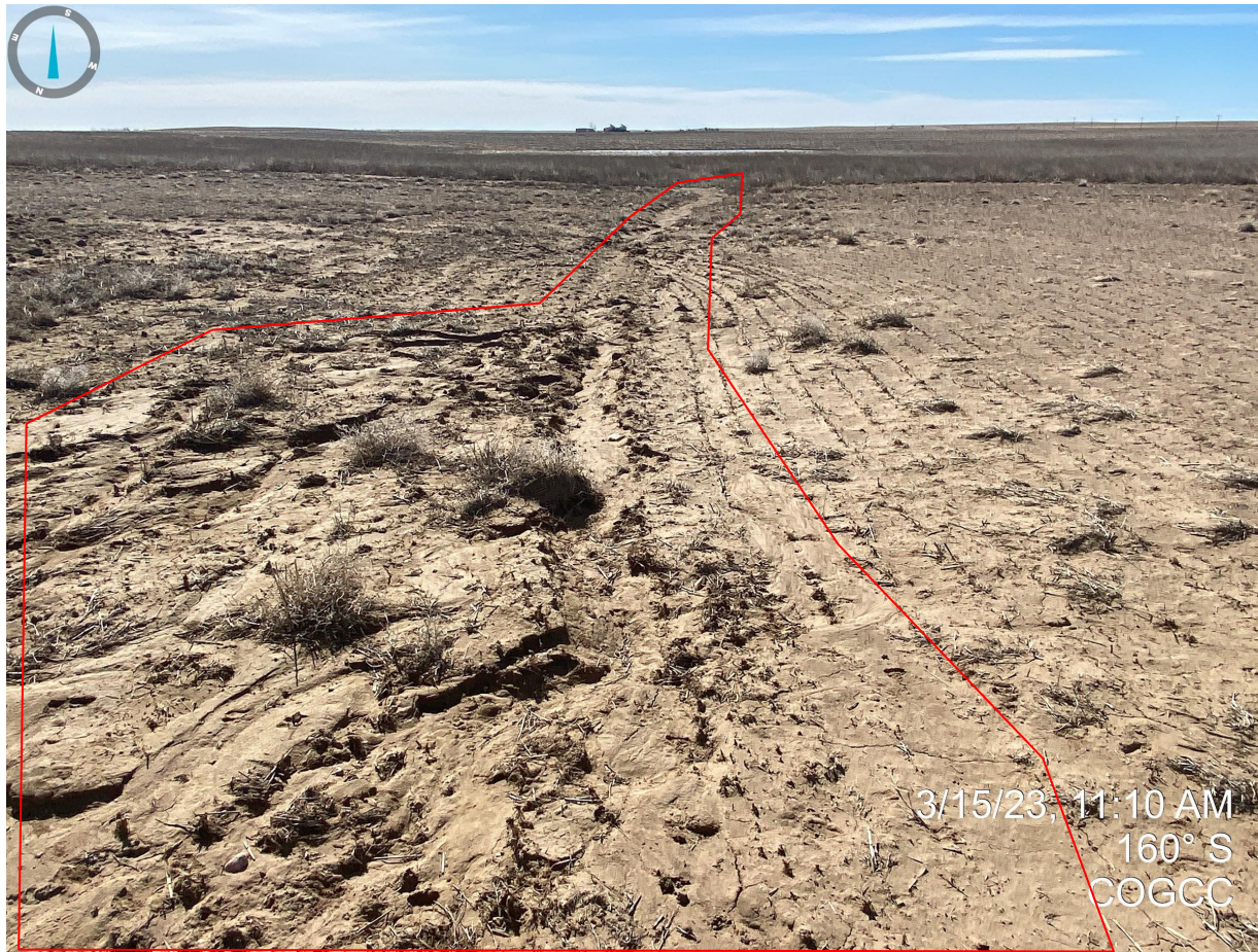
Photo 12. Facing south within recently reclaimed portion. Outline illustrates that the eroded areas have not been repaired/stabilized and no evidence of stormwater BMPs observed to prevent further off-location sediment transport. The impacted areas will need to be reclaimed, including any off-location disturbances.
