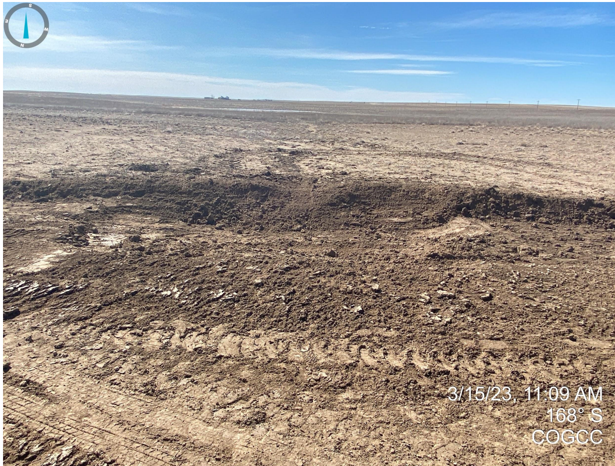
Photo 11. Facing south at sediment trap. The sediment trap does not appear stabilized at the inlet/outlets with the absence of rip-rap, erosion control blanket, etc. Additionally, the berms are comprised of loose/unconsolidated material and need to be properly stabilized to prevent further off-site sediment transport.
