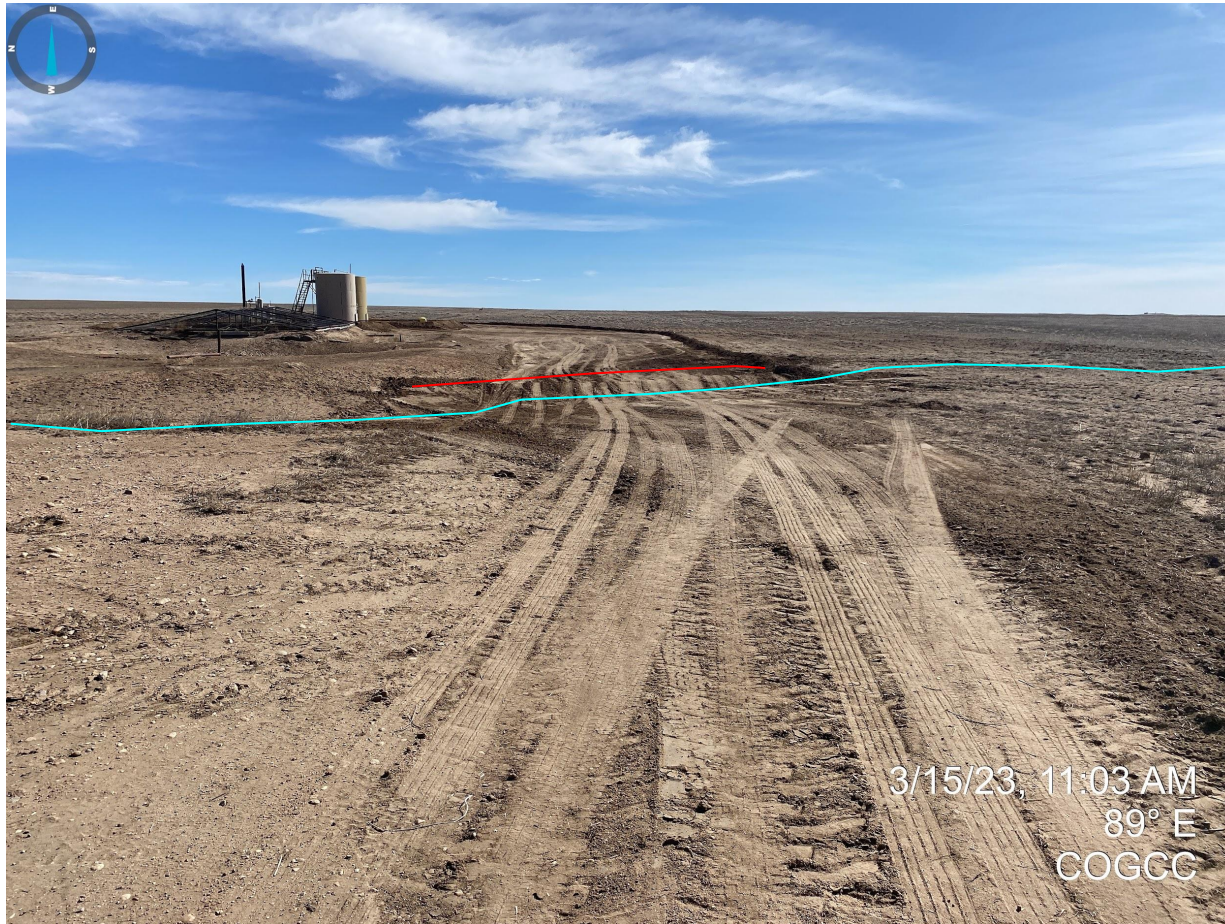
Photo 1. Facing east towards location. A water bar (red line) was constructed that appears will divert any stormwater run on/off through the location and towards the eroded area. Blue line illustrates the potential path of stormwater travel with current BMP in place.
