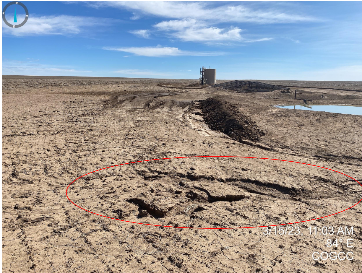
Photo 5. Facing east from the northwest corner of the location. Photo illustrates the eroded areas have not been stabilized and no BMPs were observed to prevent further stormwater erosion from occurring.
