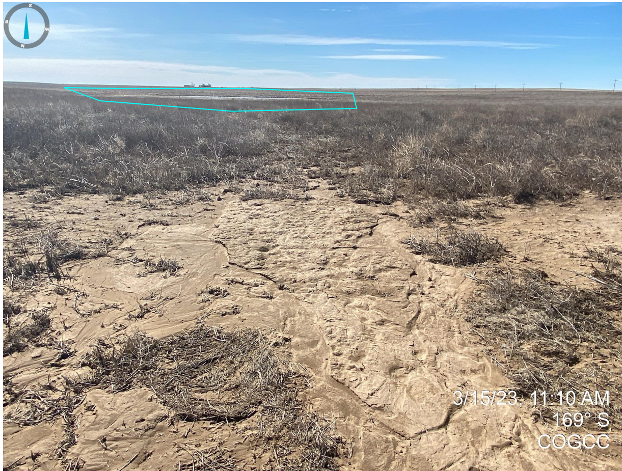
Photo 14. Facing south at adjacent land. No stormwater BMPs were identified at the time of this inspection that would prevent sediment laden stormwater from continuing to exit off location. Blue polygon illustrates freshwater emergent wetland approximately 600' south and down gradient of location. This portion of disturbance will need to be reclaimed per Rule 1004.
