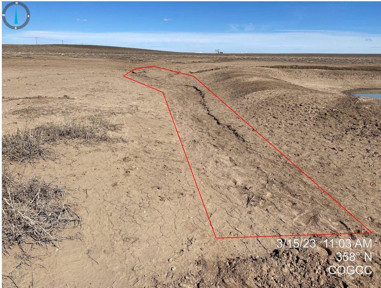
Photo 2. Facing north near the eroded area next to pit. No BMPs were observed to prevent or manage stormwater run on and run off with evidence of rill erosion occurring on pit walls (red outline). This area will need to be properly stabilized to prevent further erosion from occurring.
