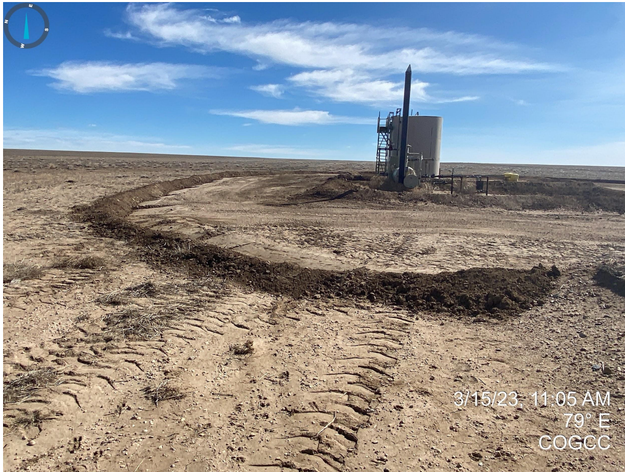
Photo 6. Facing east from the northern portion of the location. A perimeter ditch and berm was constructed around the production area; these BMPs are not sufficient as the berm material is not stabilized and is comprised of loose/unconsolidated material that can become a potential source of pollution itself.
