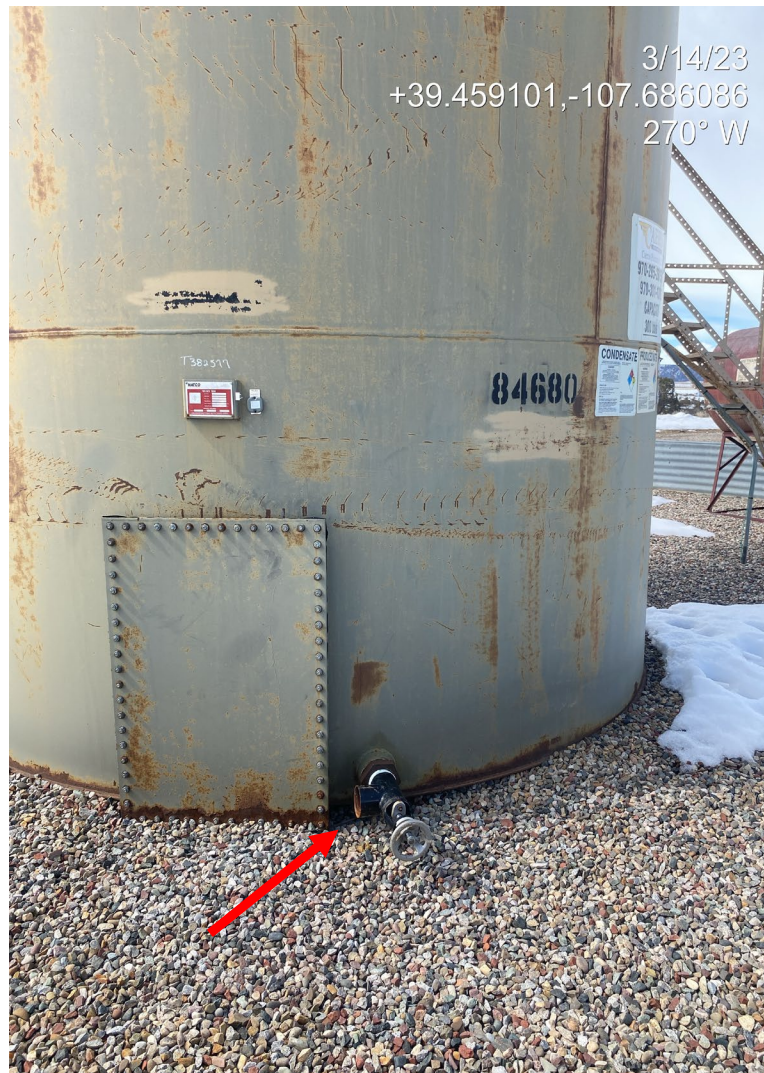
Photo 3. Photo shows a drain line without a bull plug installed.
