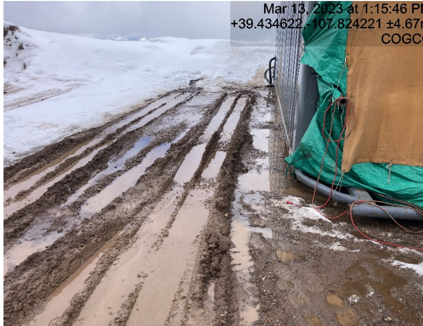
Location and lack of stabilization/compaction
