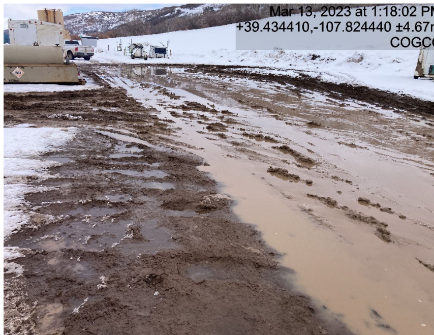
Location and lack of stabilization/compaction
