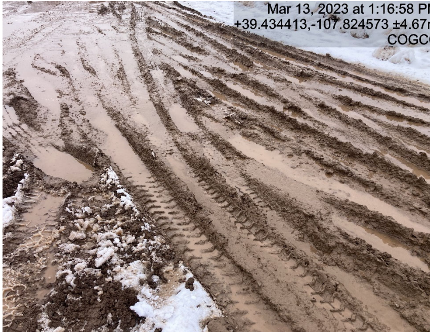
Location and lack of stabilization/compaction
