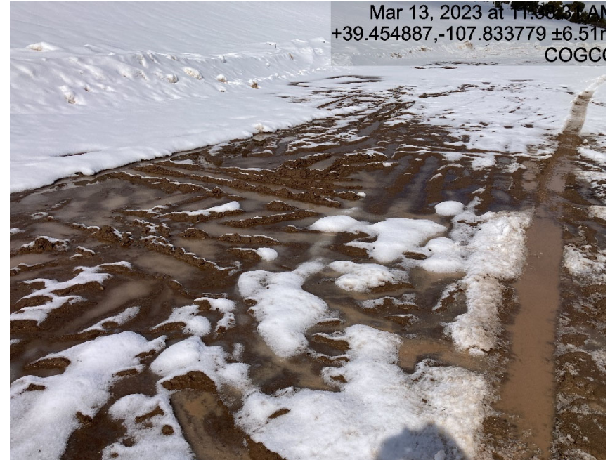
Lack of stabilization/compaction
