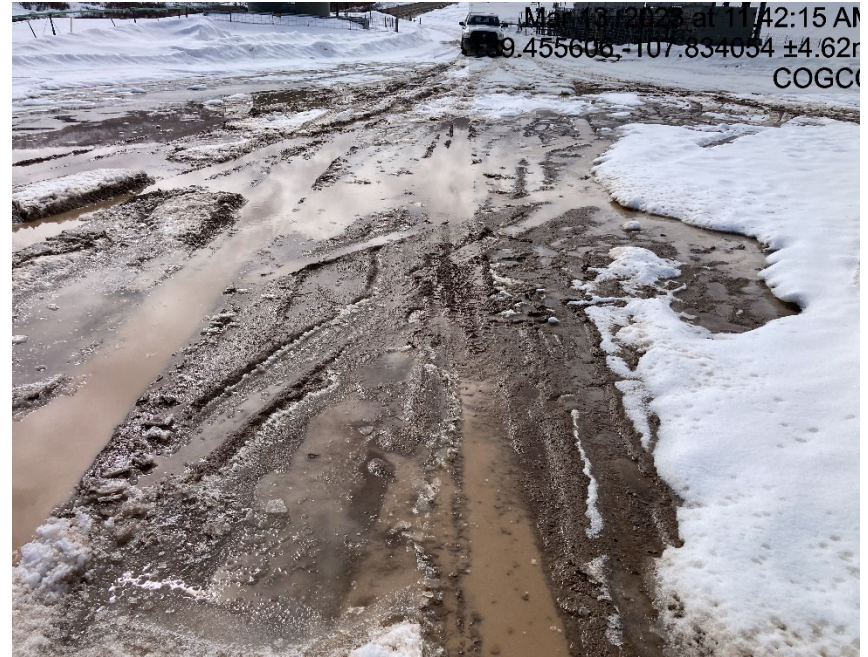
Lack of stabilization/compaction
