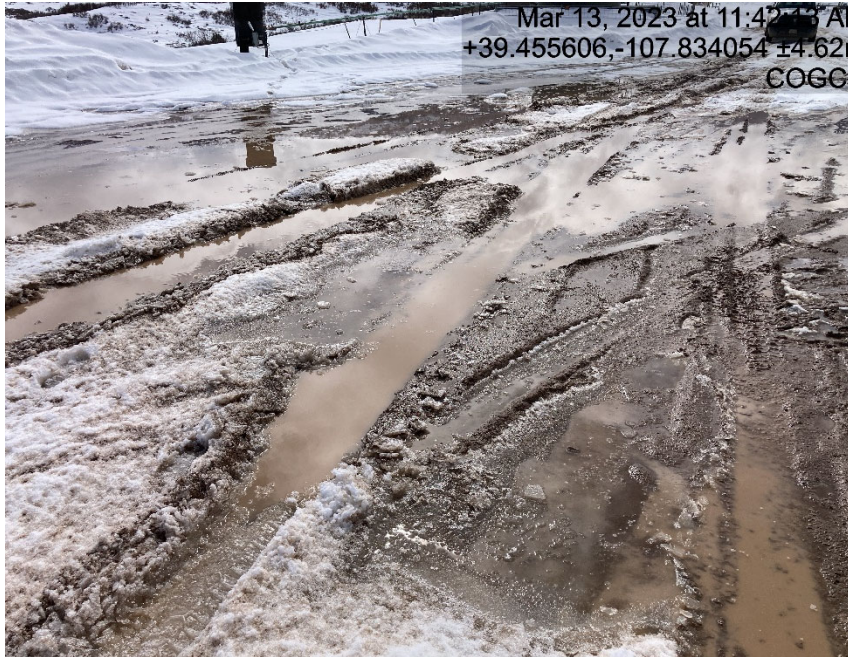
Lack of stabilization/compaction
