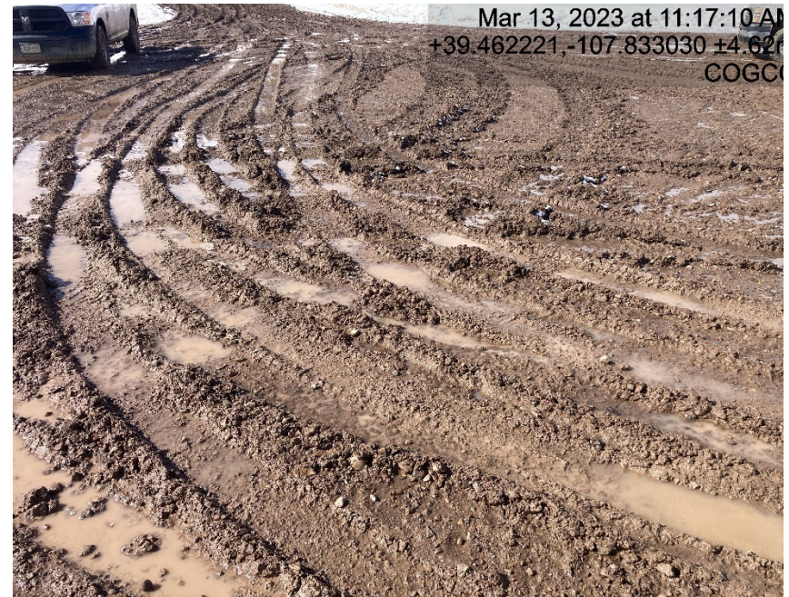
Location shows signs of lack of stabilization/compaction
