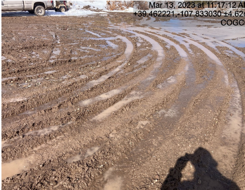
Location shows signs of lack of stabilization/compaction
