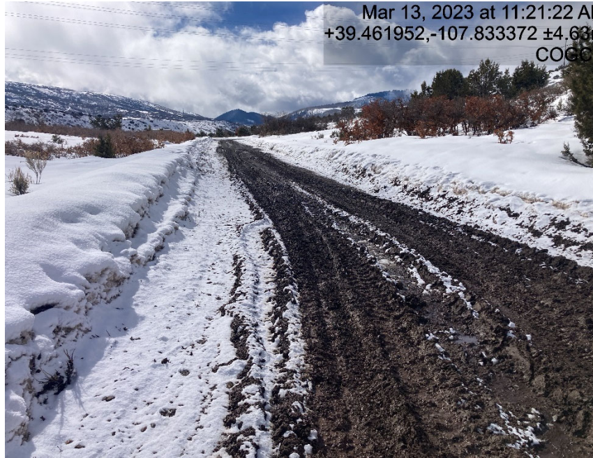
Access road lack of stabilization with sediment migration
