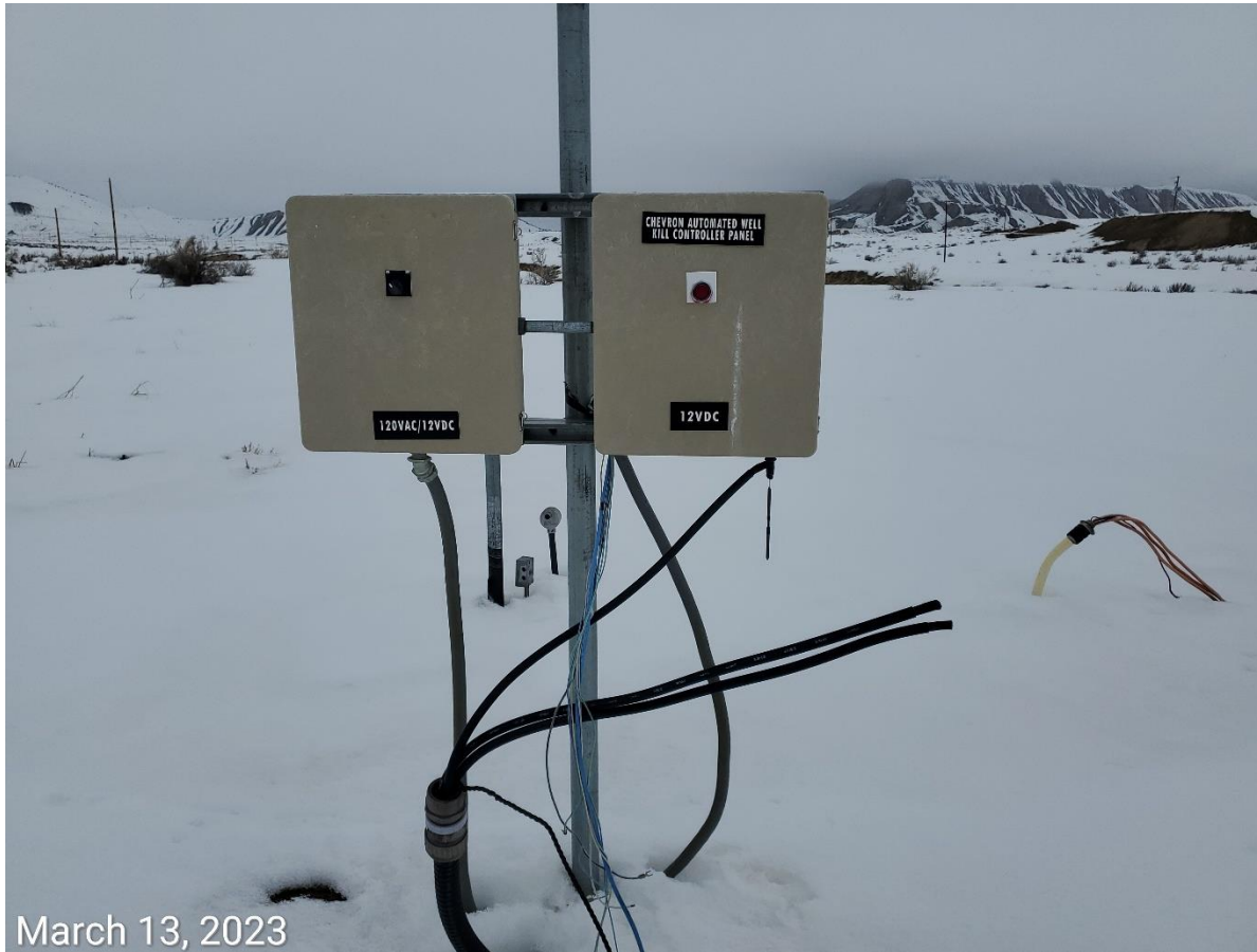
Photo 3: Electrical utility equipment has been disconnected and/or removed from the Location.
