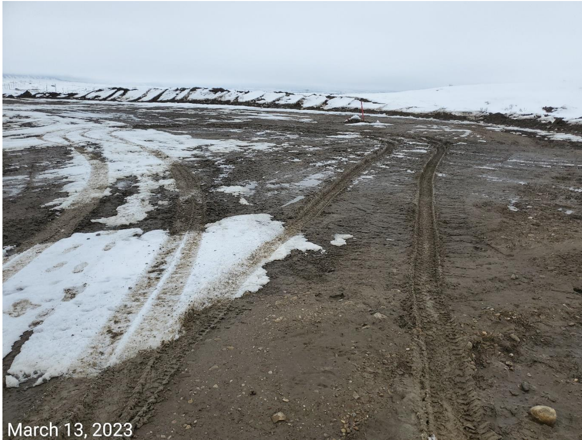
Photo 2: Tracking controls missing or insufficient.
