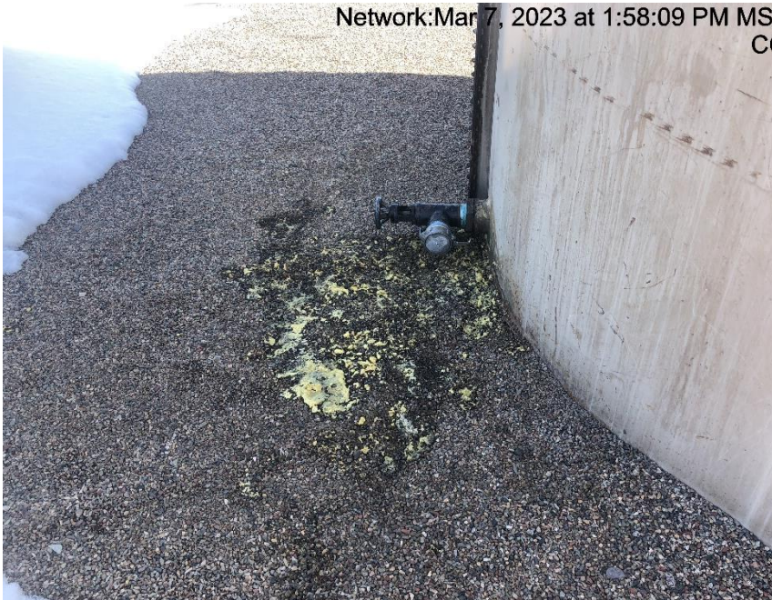
Photo #9149 Stained soils in tank containment.
