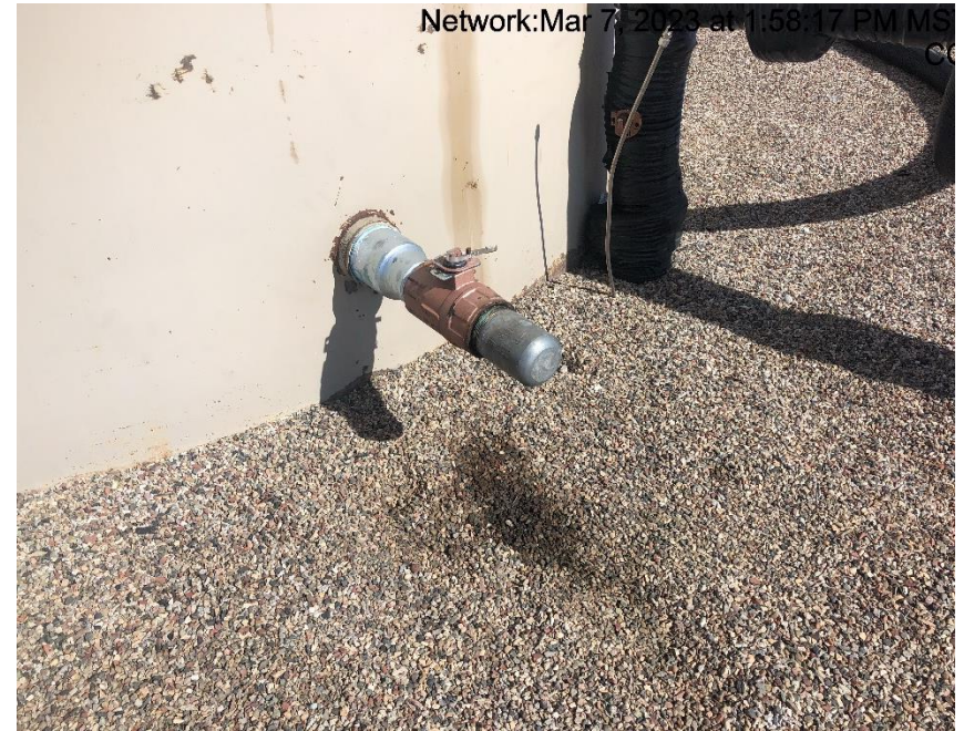
Photo #9150 Stained soils in tank containment.
