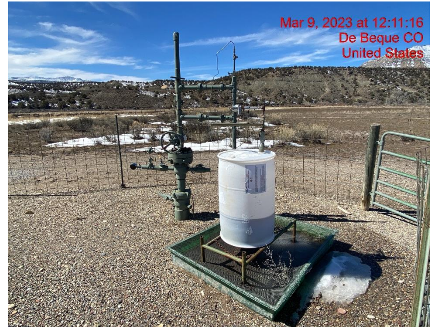
Wellhead/Chemical Tank – Photo #01309
