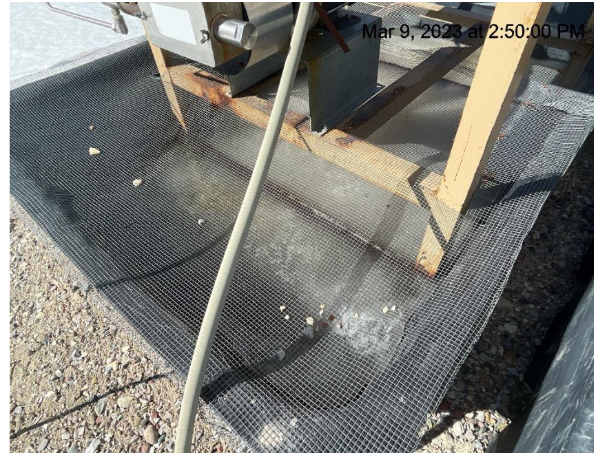
Photo # 2142 Chemical BMP not maintained
