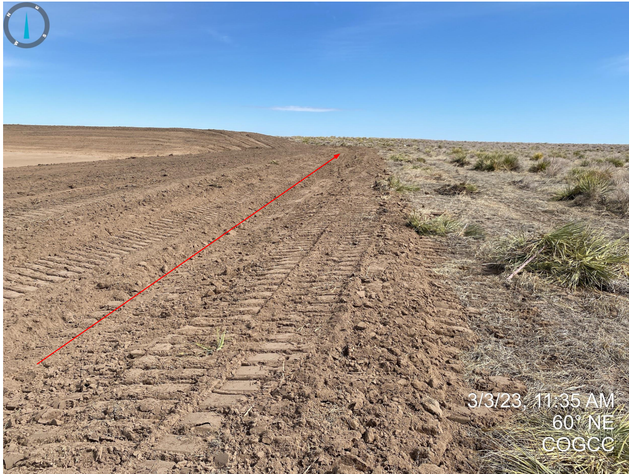
Photo 6. Facing northeast from the southwest corner of the disturbance are. Perimeter ditch and berm highlighted in red.
