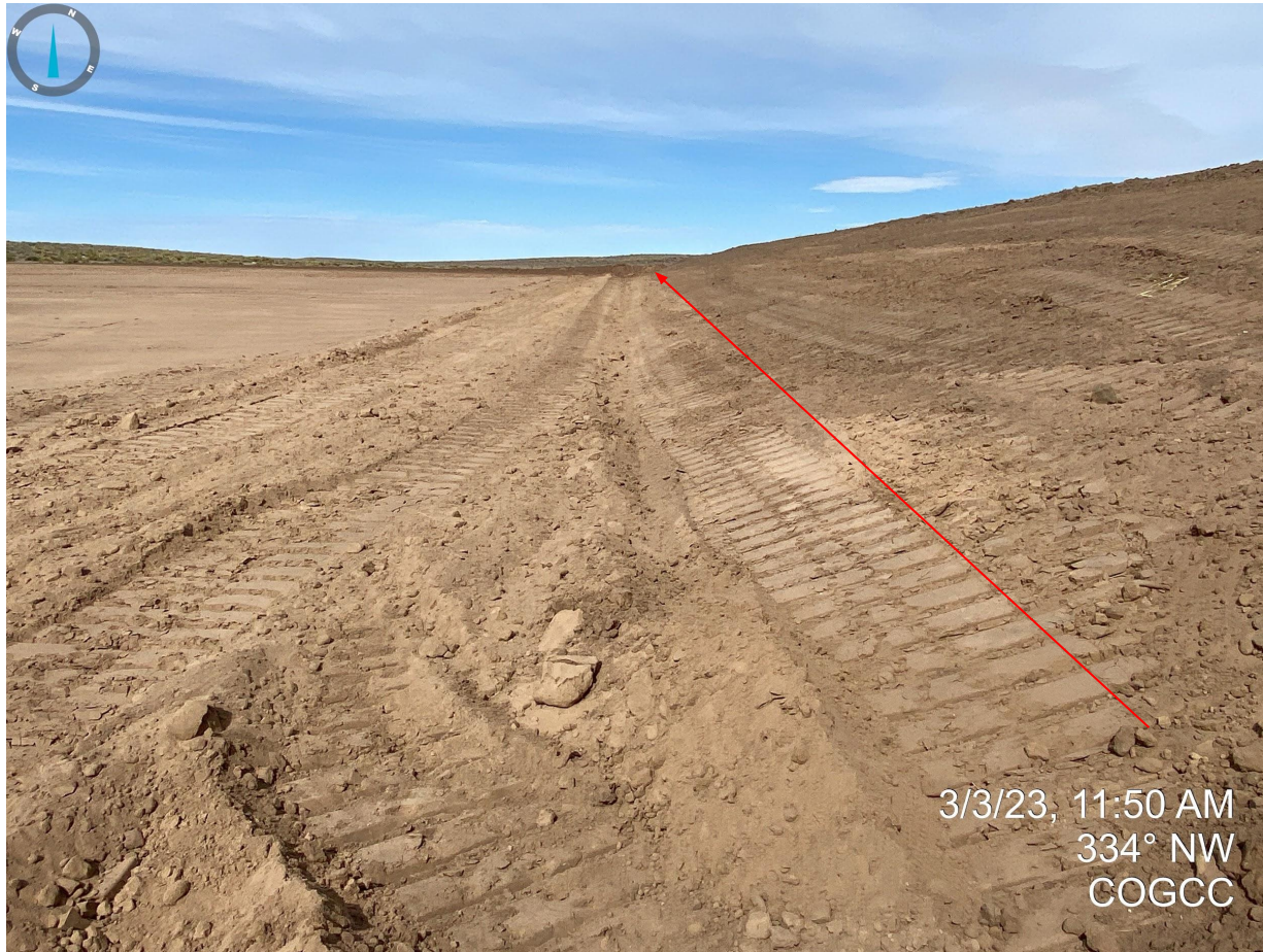
Photo 11. Facing northwest from the southern end of the topsoil stockpile. It appears the operator has salvaged all topsoil from the location with a noticeable change in soil layers observed, highlighted in red.
