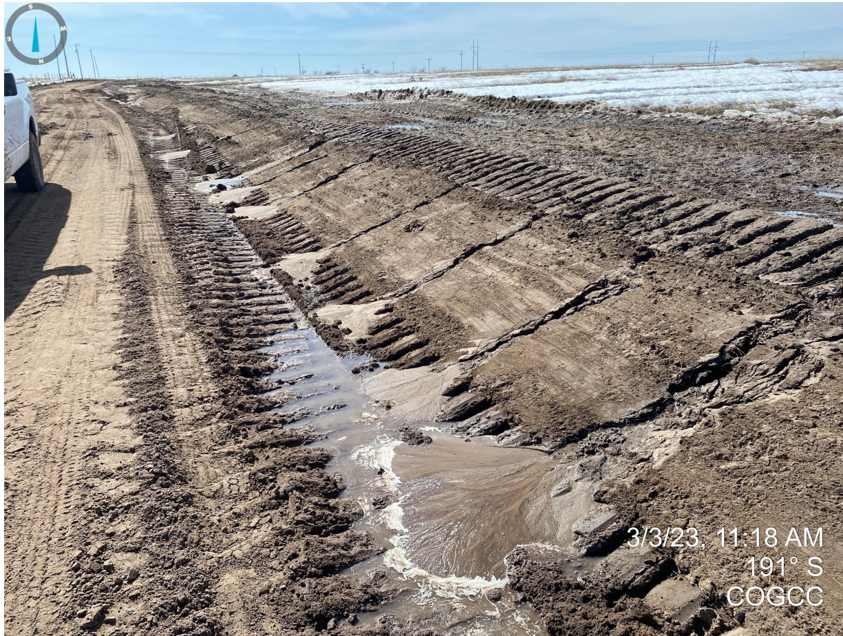
Photo 2. Facing south, approximately ¼ mile from the location's entrance, west side of road. Photo illustrates rill erosion on side of stormwater ditch and berm. This BMP will need to be repaired and maintained in accordance with Rule 1002.f.
