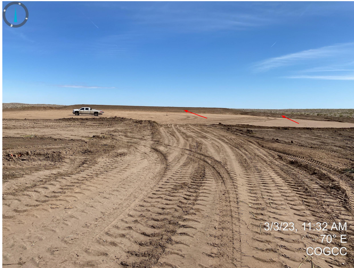
Photo 3. Facing east towards well location/pad. It appears the operator has removed all topsoil and stockpiled on the eastern and southern portions of the pad, pictured in background.
