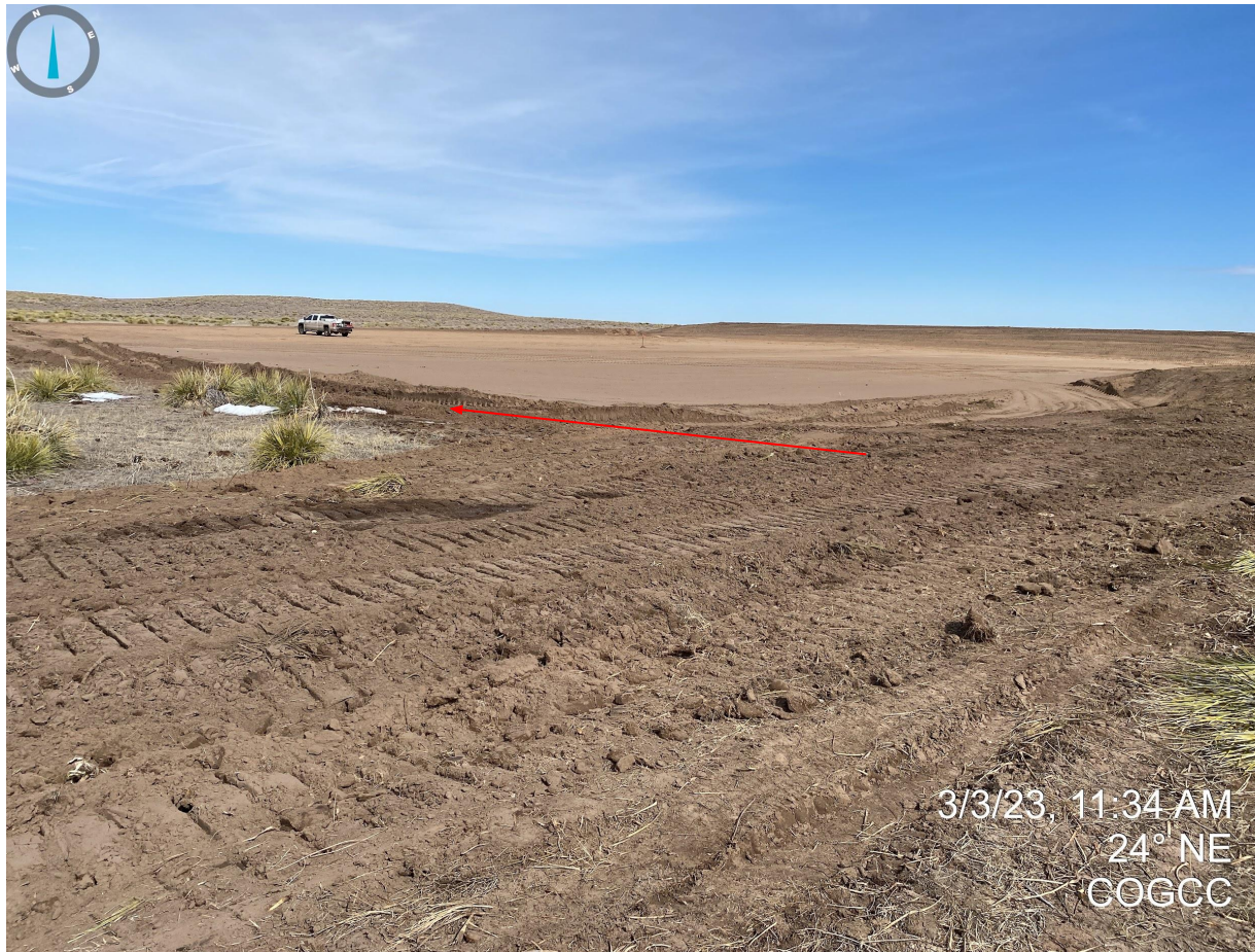
Photo 4. Facing northeast from the southwest corner of the disturbance area. Perimeter ditch and berm pictured in foreground. At this time, dirt contractors were still in the process of building the sediment trap, highlighted in red.
