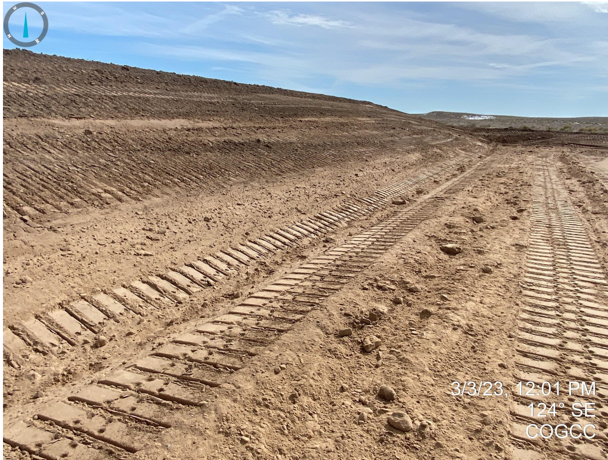
Photo 12. Facing southeast from the center (western side) of the topsoil stockpile. The stockpile has been temporarily stabilized with equipment tracking. The topsoil stockpile will need more permanent stabilization as equipment tracking is only a temporary solution. Note: equipment tracking should be perpendicular to grade to prevent soil migration from stormwater events.
