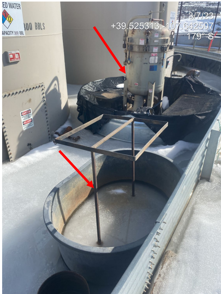
Photo 3. Photos show storage of supplies/unused equipment within the tank battery secondary containment (left) and debris, (right) including electrical equipment in disrepair within a puddle.
