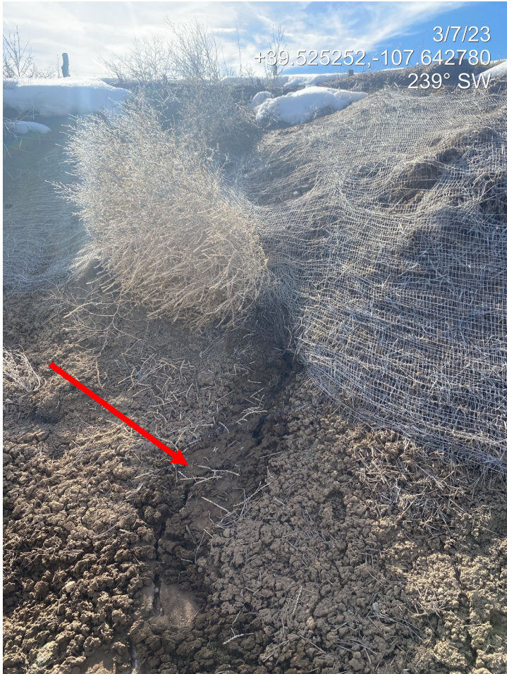
Photo 4. Photos shows the cut slope to the south of the location. BMPs (erosion control blankets) are in disrepair and are degrading. Erosion is evident. Note rill erosion (left) and sediment accumulation at the base of the cut (right) indicating loss of soil from the slope.
