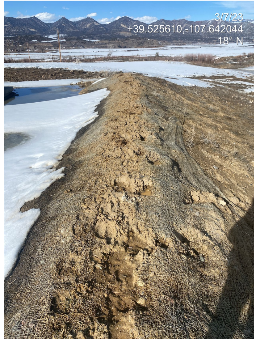
Photo 5. Photos show eastern interim areas/slopes. No perennial vegetation observed. Bare ground and annual species dominate. Stormwater BMPs have only been installed on a small portion of the slope are in disrepair. Soils are bare, unprotected.
