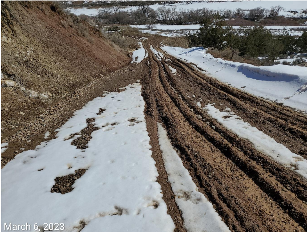
Photo 3: Photos 3-8 examples showing BMPs to manage runoff, minimize degradation, tracking and sediment transport are missing or insufficient at the access road.
