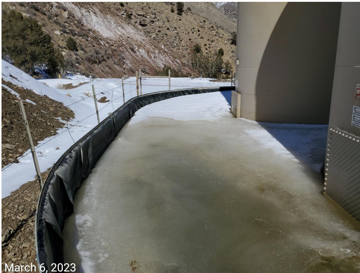
Photo 2: Photo shows secondary containment BMPs at the tank battery has filled with fluids/ice, and does not appear adequate to contain a spill.
