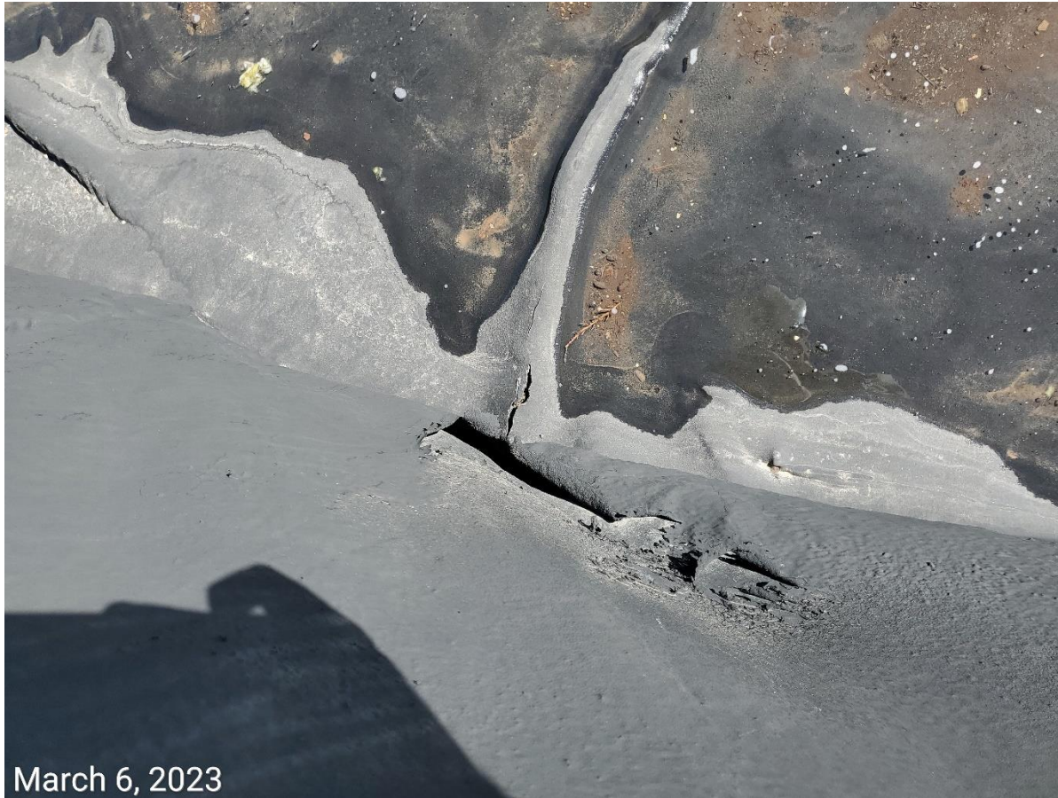
Photo 2: Cracks observed in liner.
