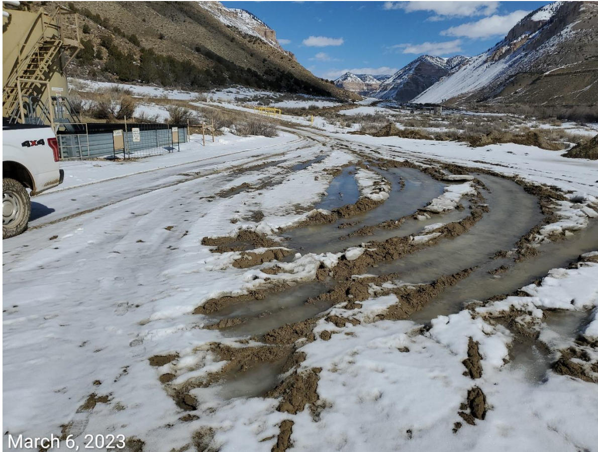
Photo 6: Photo example showing BMPs to minimize tracking and degradation are missing or insufficient on the Location.
