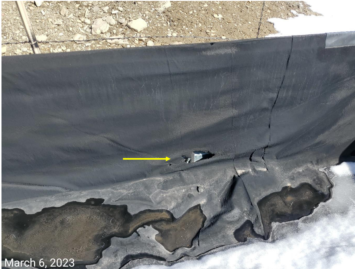
Photo 1: Photo example showing liner integrity at the tank battery remains compromised.
