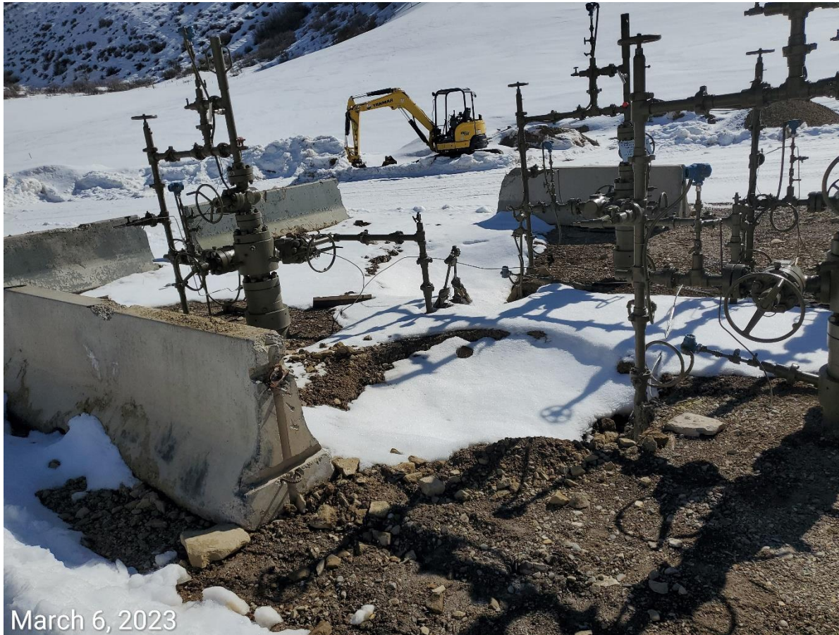
Photo 1: Conductor plugging/reclamation “in process”.
