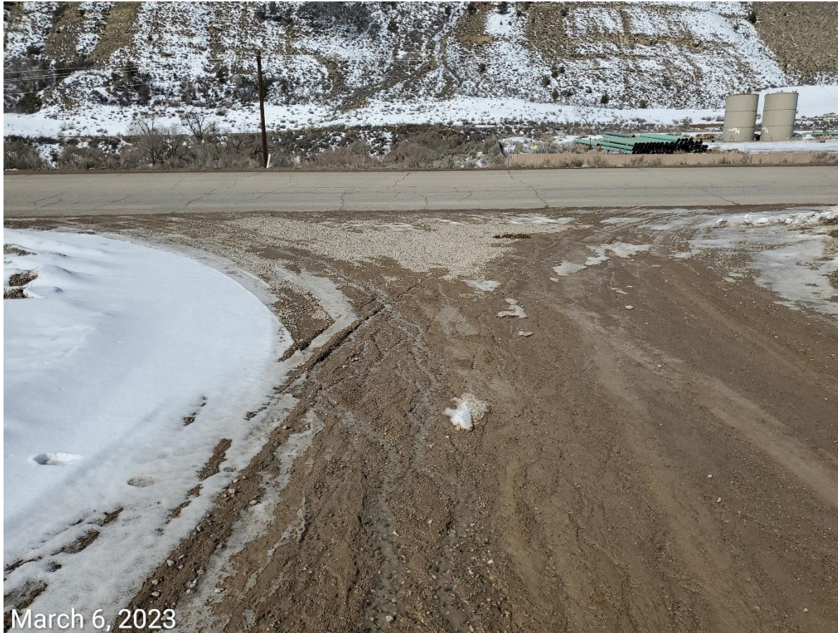
Photo 5: BMPs along access road showing signs of disrepair. Maintenance advised prior to failure of BMP.
