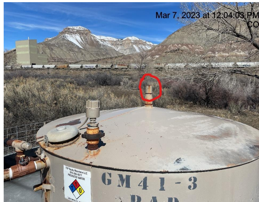
Photo # 1808 Open ended pipe on production tank
