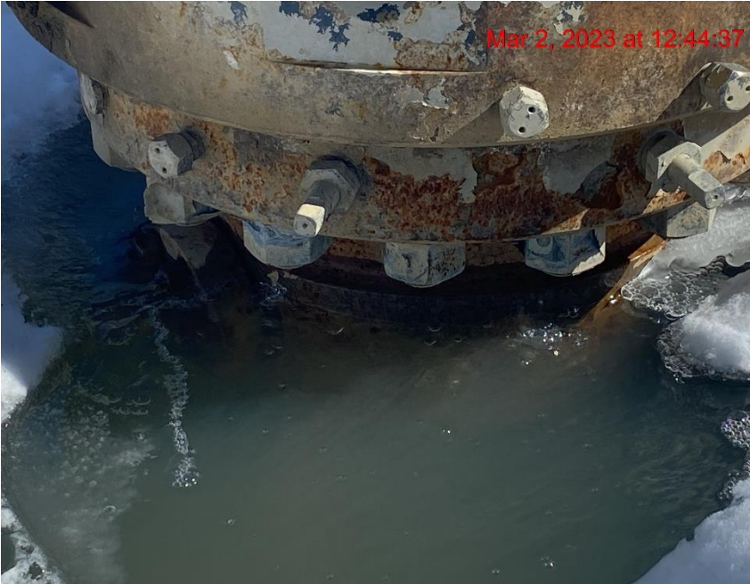
Casing Flange Leak (Bubbling) – Photo #01117
