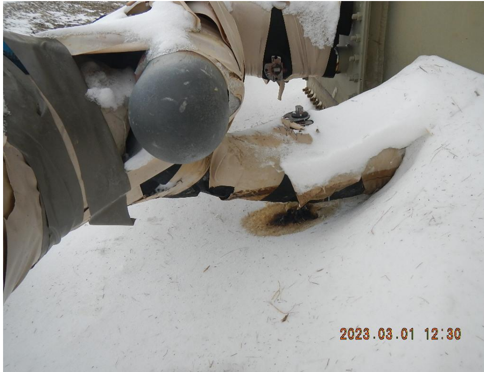
Photo 2. Valve leaking on middle easternmost Produced Oil tank.
