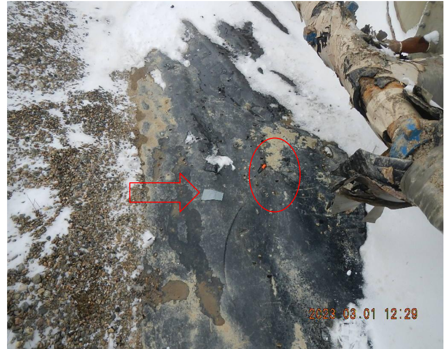
Photo 5. Liner with holes and repair. Note: Arrow points to Duct Tape repair. Circle depicts pen through liner penetration
