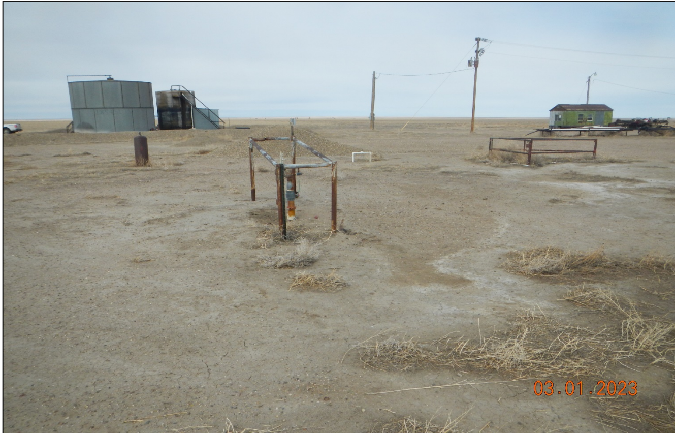
Photo 6. South side of the location facing north at the location. There are unmarked pipe risers at this side of the location which should be removed.
