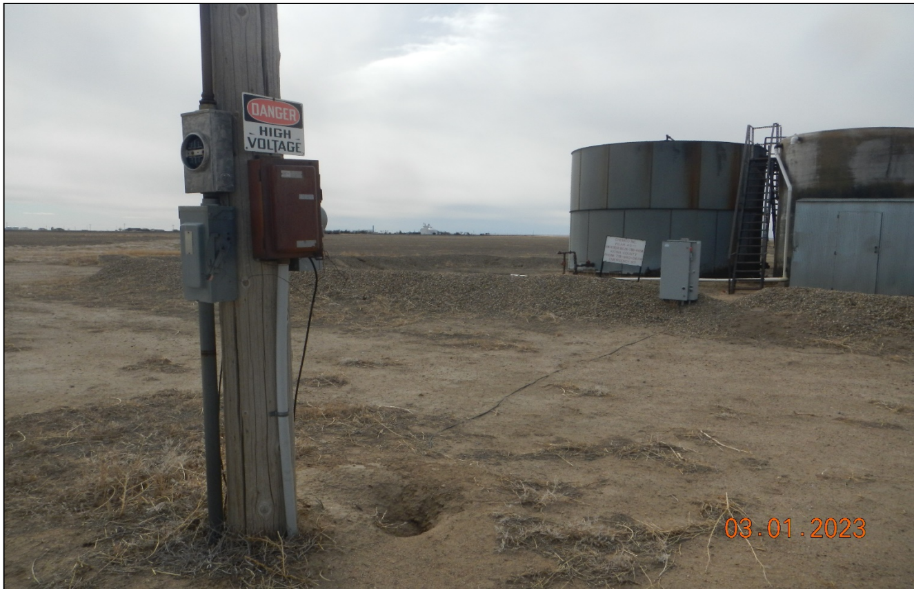
Photo 12. There is an electric wire on the ground which can be a safety issue as it is not properly protected. Sign is posted at the battery.
