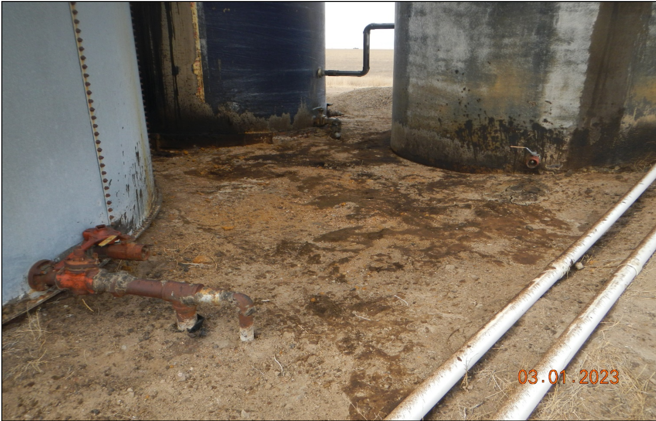
Photo 4. There is oil staining around the tanks which needs to be cleaned up.
