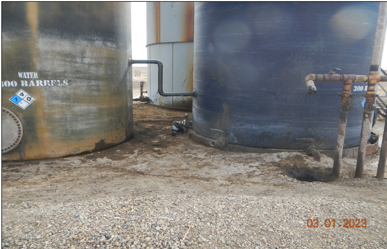
Photo 2. There is oil stained soil around the tank from a spill contained inside the bermed area.
