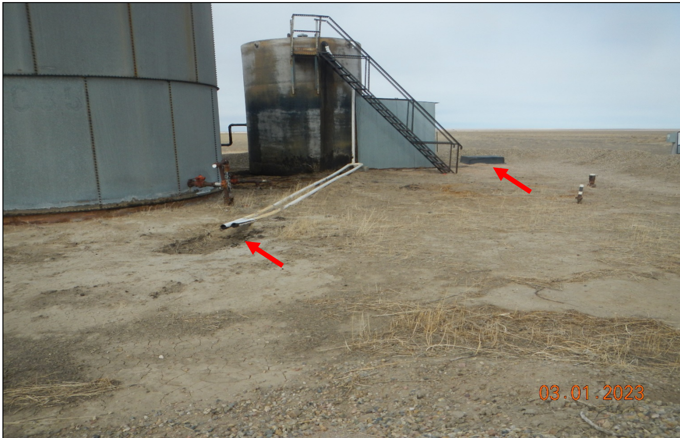
Photo 5. The container at red arrow was position to catch oily waste at the whit pipes which has been displaced.
