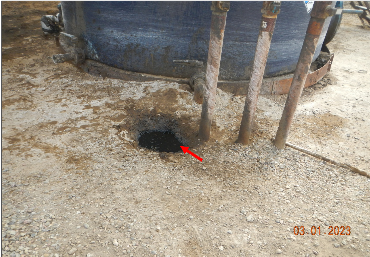
Photo 3. There is a puddle of oil which appears to be a shallow hole where oil has accumulated.
