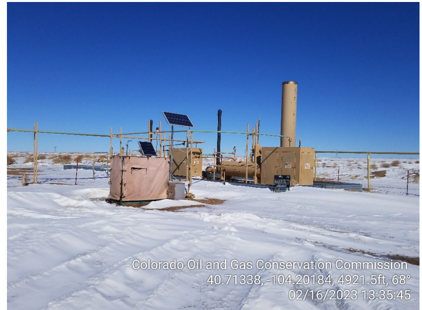
Photo 4 – Separators, VRU and ECD
