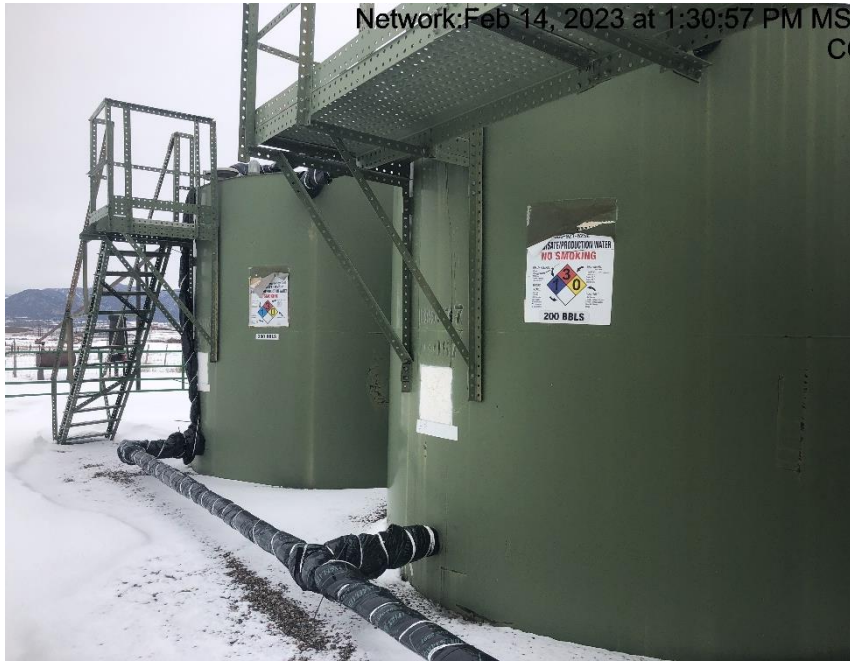
Photo #9021 Multiple tank labels weathered and not legible.
