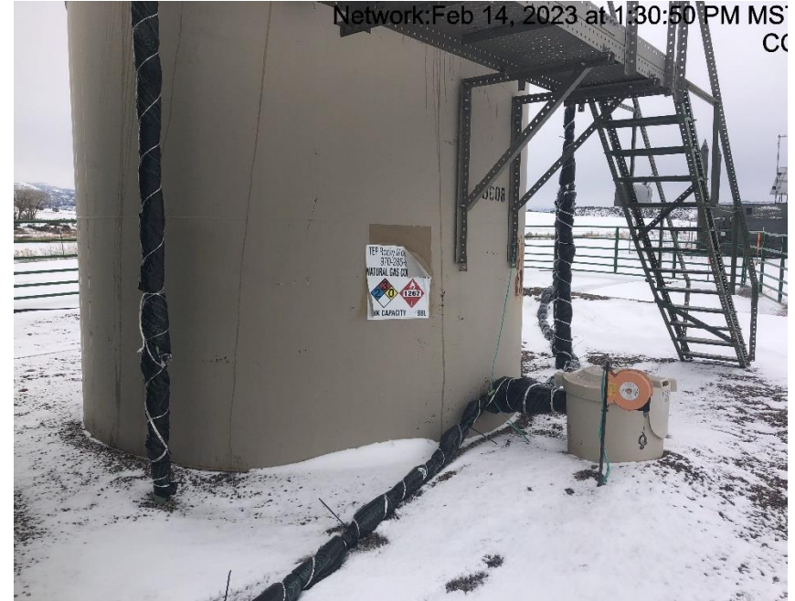
Photo #9020 Multiple tank labels weathered and not legible.
