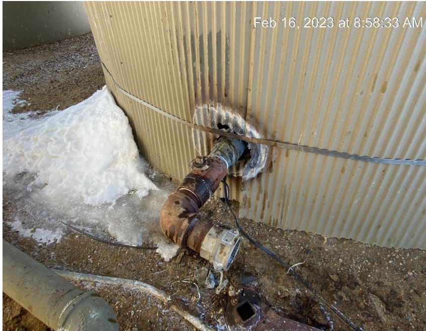
Line on tank missing cap and evidence of burn marks around pipe. Insulation is melted and tin is charred.
