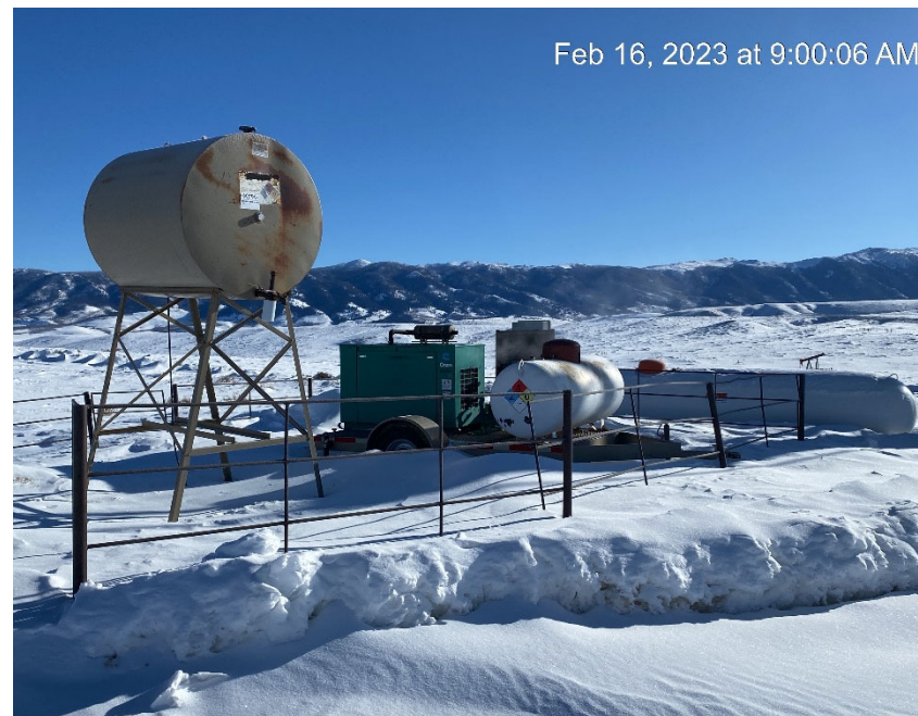
Diesel tank lacking secondary containment
